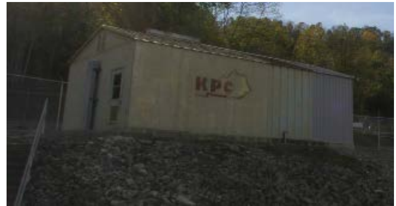
Existing Control House
