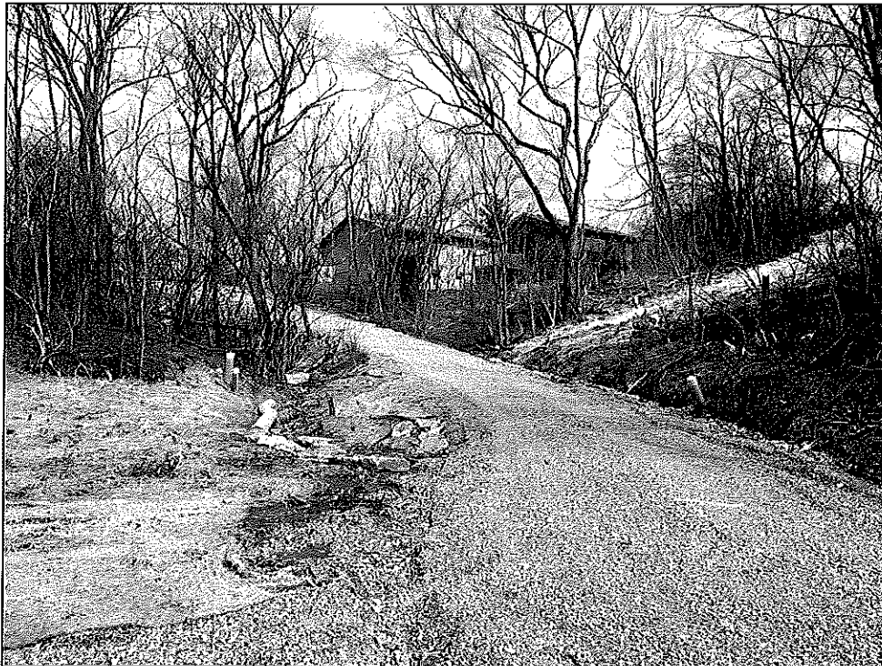
Collection line replacement
