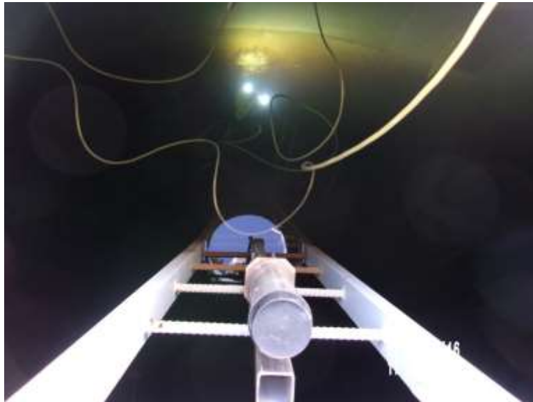
PHOTO SHOWS OPEN VIEW OF ROOF HATCH
