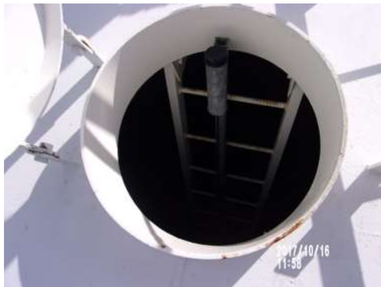
PHOTO SHOWS OPEN VIEW OF ROOF HATCH
