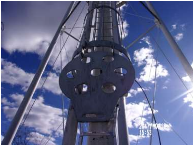
PHOTO SHOWS UPWARD VIEW OF LADDER IN GOOD CONDITION
