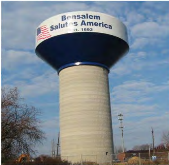
New 2 MG Tank
