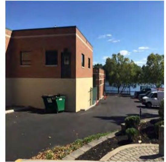
Bristol WTP Expansion
