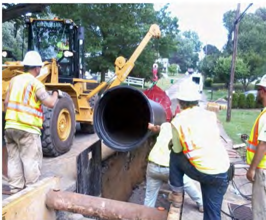
Water Main Reinforcement
