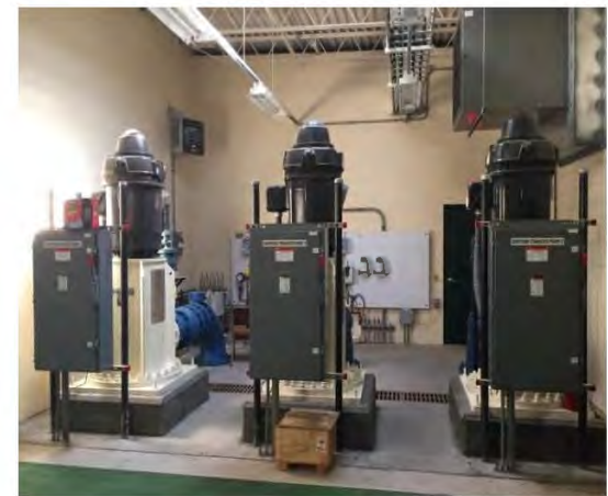
Bristol Booster Replacement
