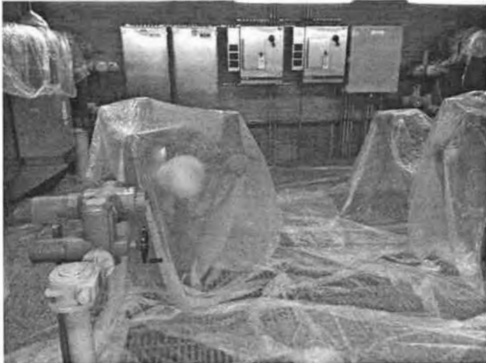
Rehabbed Valve Room At Kentucky River Station I Water Plant
