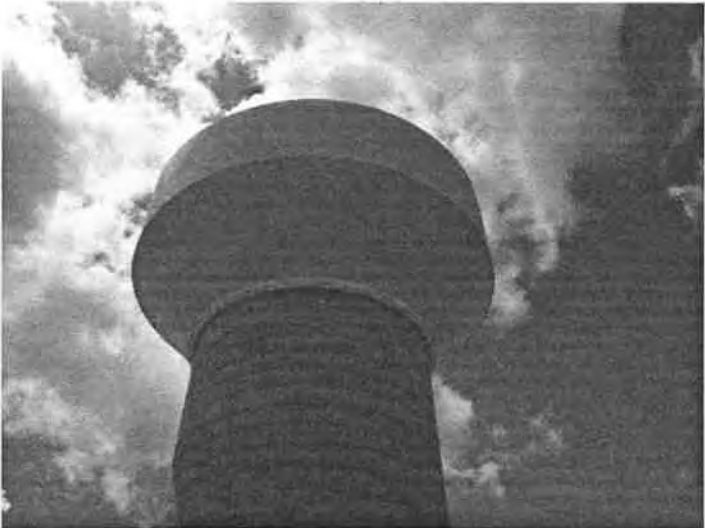
Eastland Water Storage Tank
