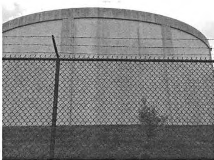
Clay's Mill Water Storage Tank 2
