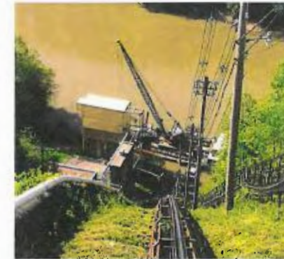
Figure 2: Barge Unloading at Raw Water Intake Structure
