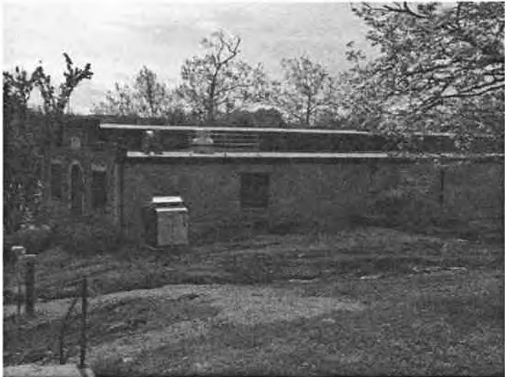
Richmond Road Water Treatment Plant Old Filter Building
