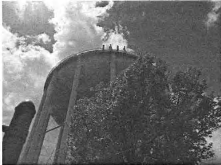
Parkers Mill Water Storage Tank
