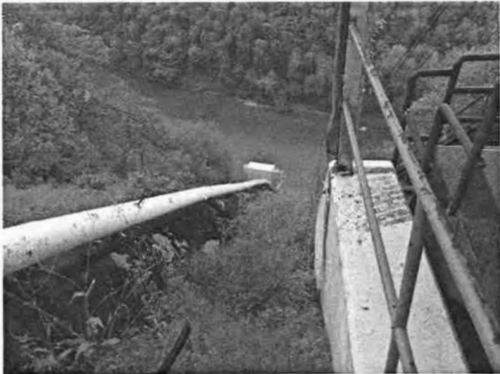
Raw Water Line at Kentucky River Station I Water Treatment Plant
