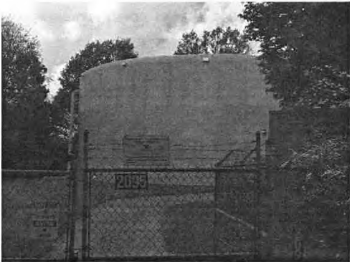
Clay's Mill Water Storage Tank 1
