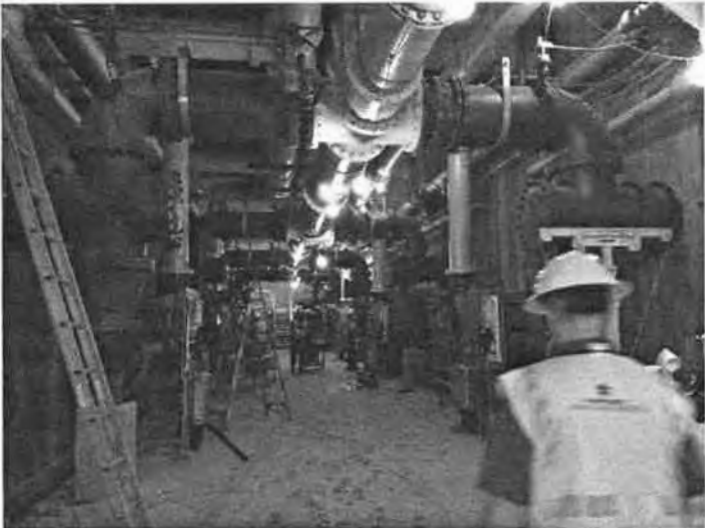
Pipe Gallery at Richmond Road New Filter Building
