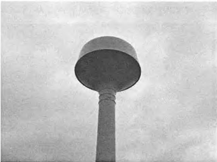
Fair Grounds Water Storage Tank
