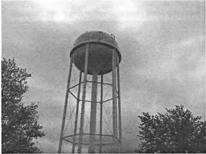
Blue Moon Water Storage Tank
