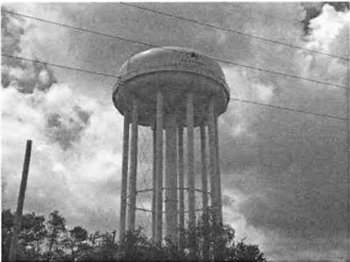
Cox Elevated Water Storage Tank
