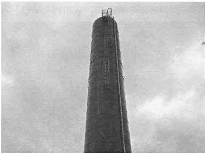
Bromley Water Storage Tank
