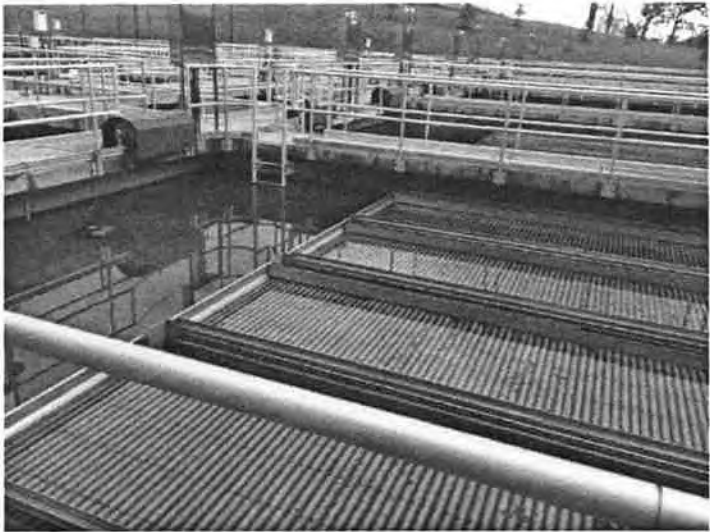
Settling Basin at Kentucky River Station II Water Treatment Plant
