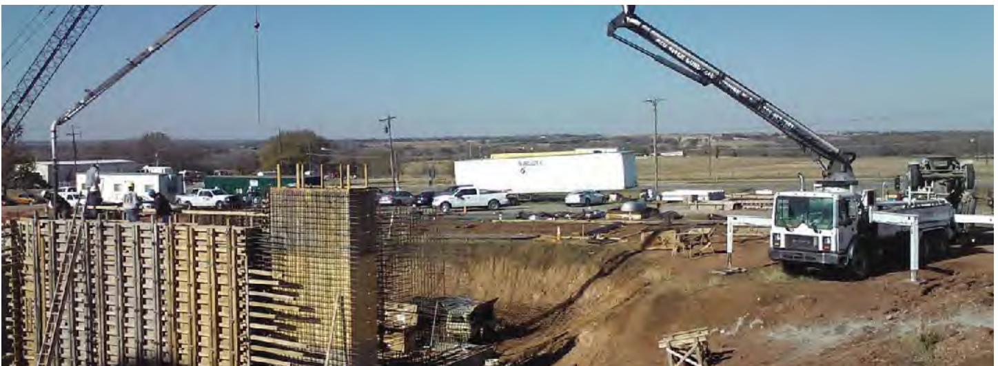
Super Pulsator Water Treatment Plant at the Davis Municipal Authority in Oklahoma.
