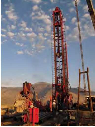
John Taylor, Farr West Engineering Construction of new municipal well in Hawthorne, NV.
