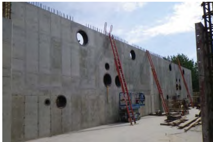
Chad Kolstad, Minnesota Department of Public Health New surface water treatment plant in Fairmont, MN. The current plant was constructed in 1926 and needed to be replaced. The new plant will have biologically active GAC filters to help with taste and odor complaints.
