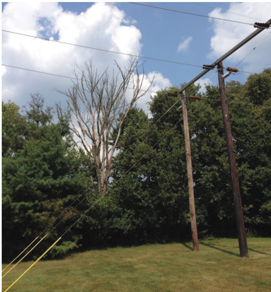
Figure 18: Example of a hazard tree adjacent to a 69kV transmission line.
