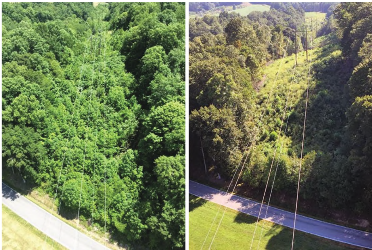
Figure 16: Before and after — example of the cleared transmission right-of-way.
