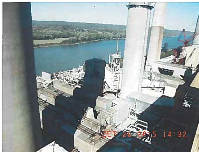
Unit 3 Scrubber at Ghent Generating Station
