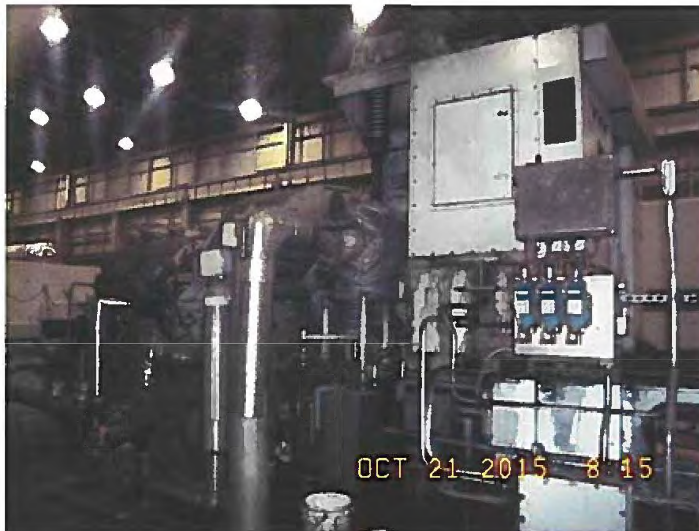
Steam Driven Boiler Feed Pump (Unit 3) at Mill Creek Generating Station
