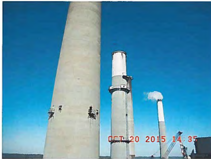
Units 1-3 Stacks at Ghent Generating Station
