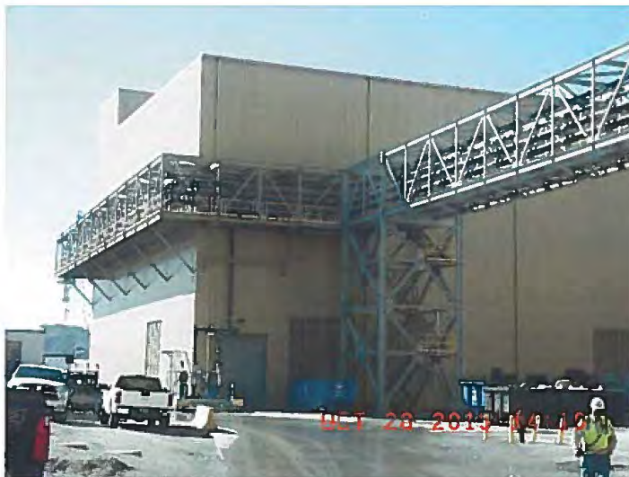
Limestone Prep Building at Ghent Generating Station
