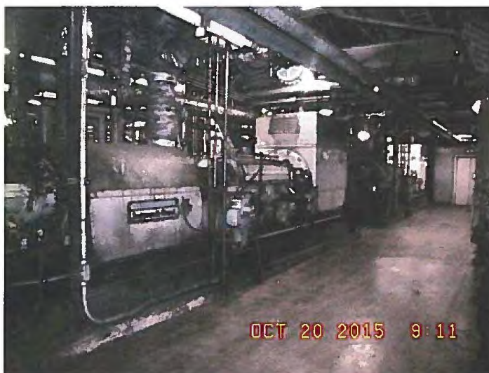
Boiler Feed Pumps at Brown Generating Station
