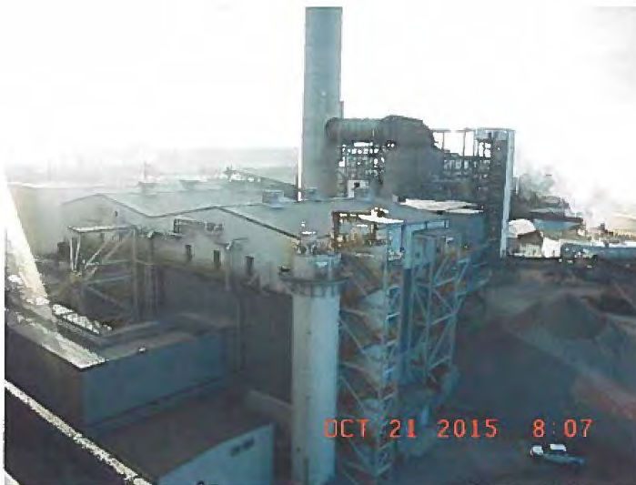
Unit 4 Scrubber at Mill Creek Generating Station
