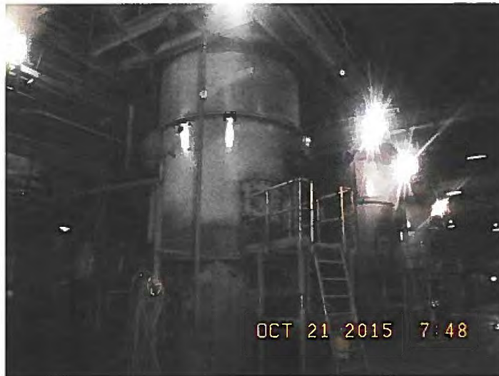
Unit 3 Pulverizers at Mill Creek Generating Station
