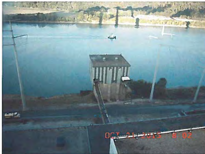
Intake at Mill Creek Generating Station
