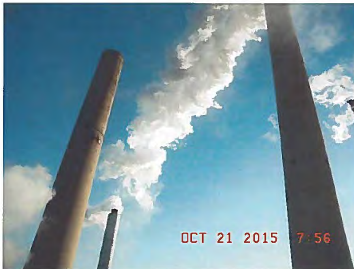
Stacks at Mill Creek Generating Station
