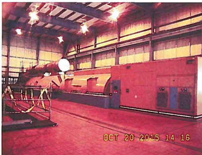
Unit 3 Turbine at Ghent Generating Station
