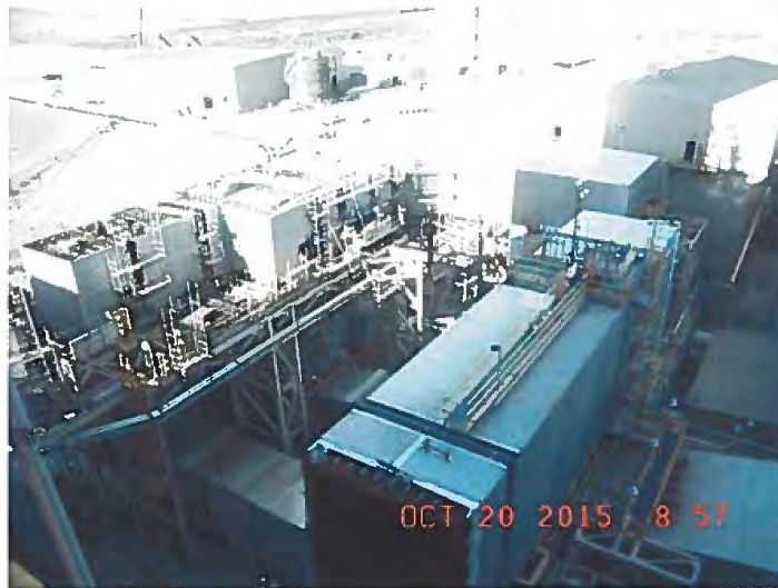
Air Exhaust/ID Fan at Brown Generating Station
