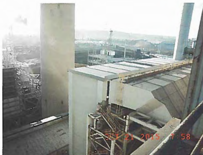
Unit 3 SCR at Mill Creek Generating Station
