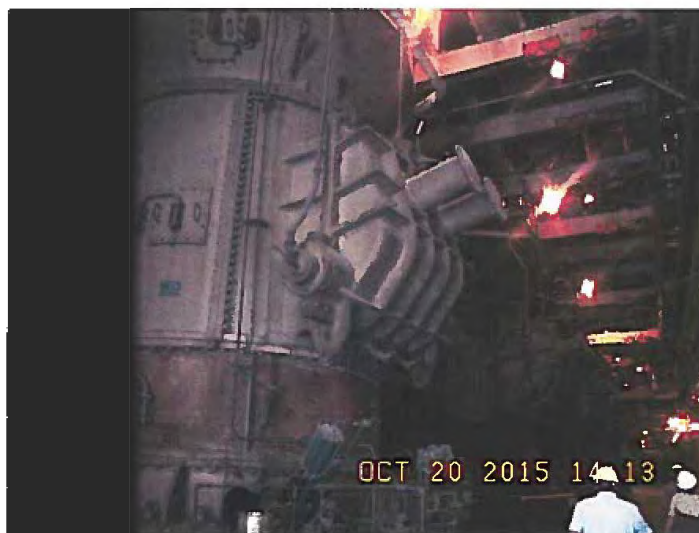
Pulverizers Unit 4 at Ghent Generating Station
