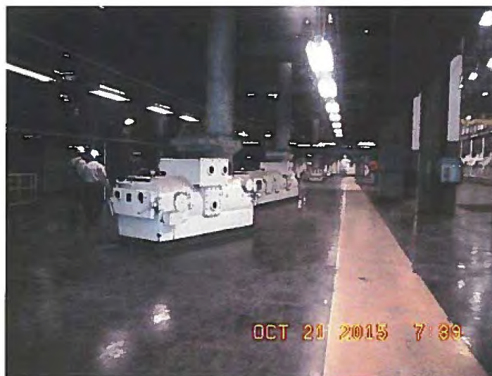
Coal Feeders at Mill Creek Generating Station
