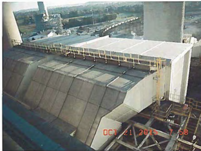
Unit 2 SCR at Mill Creek Generating Station
