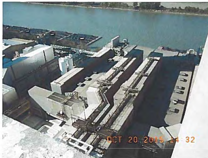
Unit 4 Precipitator at Ghent Generating Station
