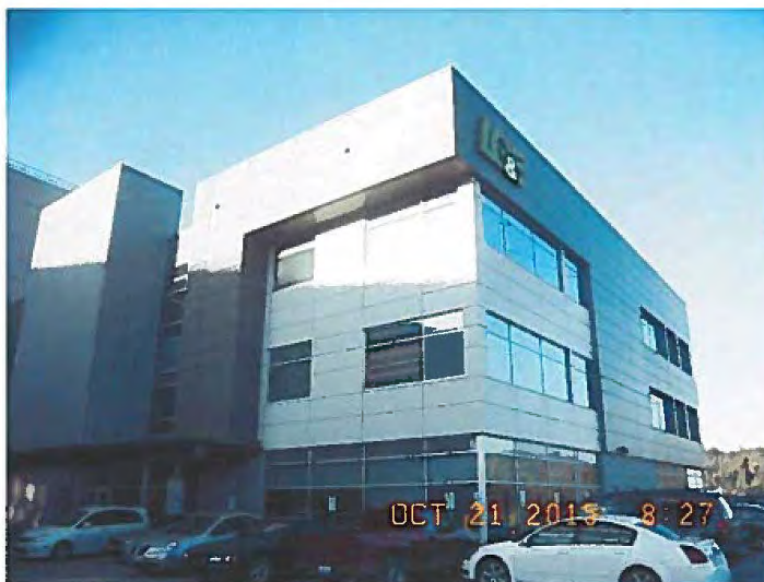
Administration Building at Mill Creek Generating Station
