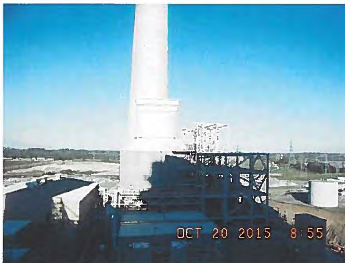
Scrubber at Brown Generating Station
