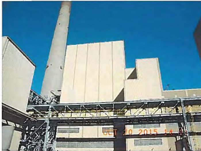
Unit 4 Boiler at Ghent Generating Station
