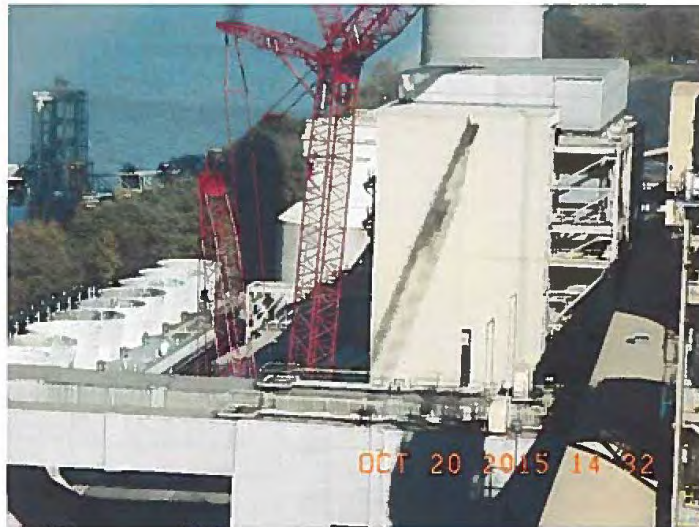
Unit 1 Scrubber at Ghent Generating Scrubber
