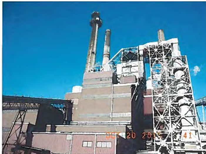
Units 1 & 2 at Brown Generating Station
