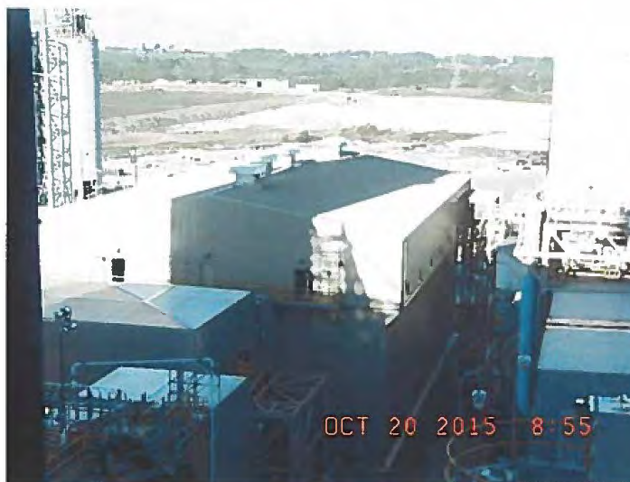
Baghouse at Brown Generating Station
