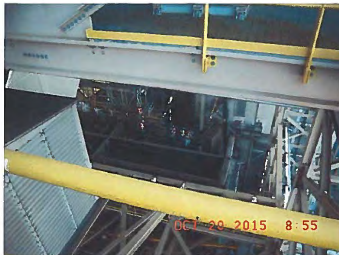
Precipitator (being demolished) at Brown Generating Station
