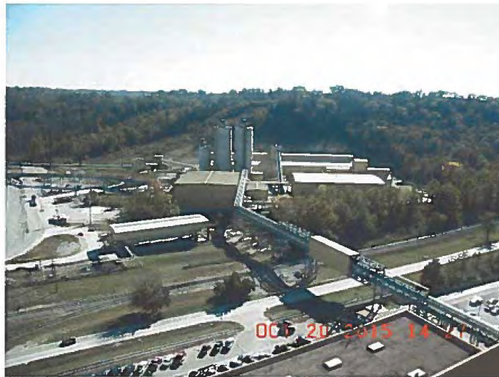
CCRT facility at Ghent Generating Station
