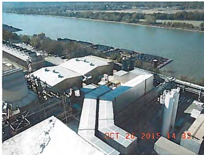
Unit 4 Baghouse at Ghent Generating Station
