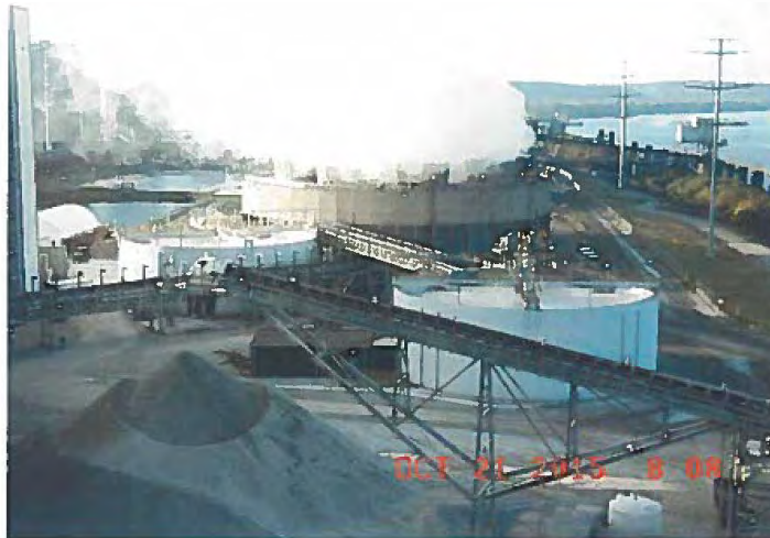
Limestone Slurry and Unit 4 Cooling Tower at Mill Creek Generating Station
