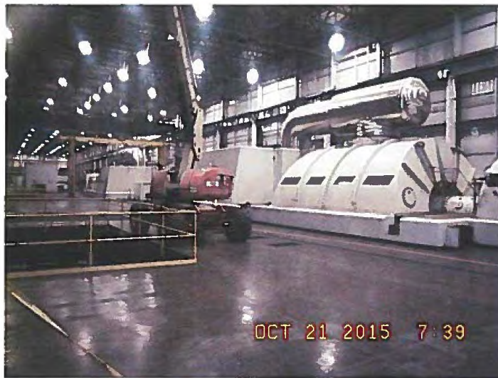
Units 1 & 2 Turbines at Mill Creek Generating Station
