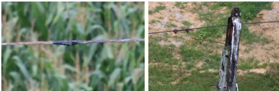
The picture on the left highlights a broken conductor strand and corrosion, which is representative of the wire condition. The picture on the right shows one of many broken grounding wires, corrosion to the static wire and ridge iron, and general degradation of the wood pole that has occurred over the asset's service life. Left unrepaired these conditions leave the system vulnerable to future unplanned outages.
