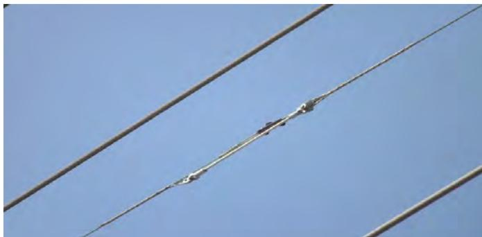
The aging static will be replaced with OPGW. In addition, new steel structures will be installed in place of existing wood structures.
