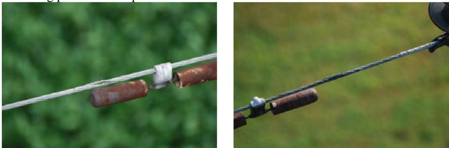
The picture on the left shows broken strands on the existing conductor and signs of corrosion on the steel core. The picture on the right highlights evidence of damage to the existing conductor, and hardware age.
