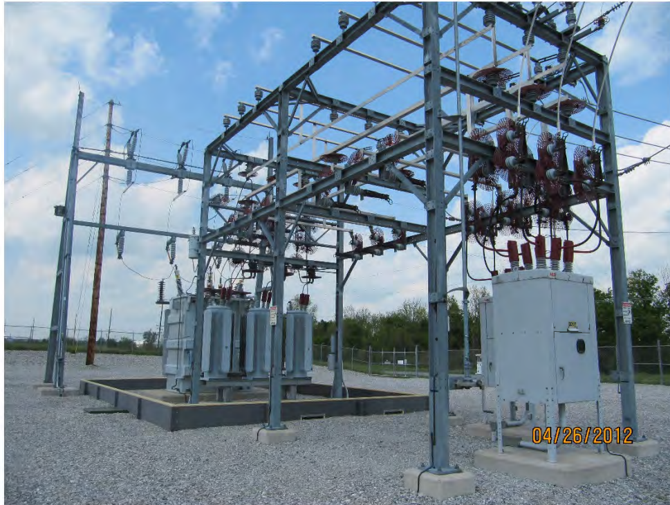
Figure 2 KU Outdoor 12kV Bus Construction
