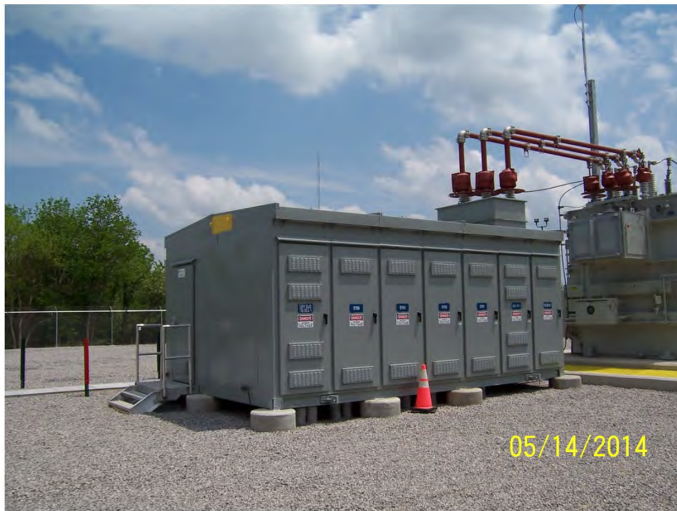
Figure 1 Metalclad Switchgear Indoor 12kV Bus Construction
