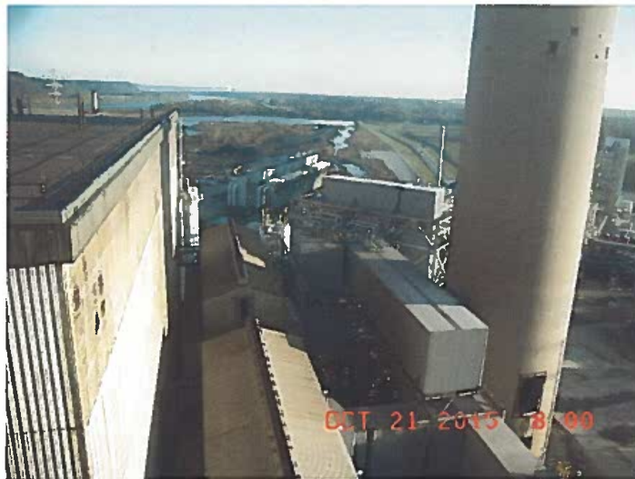
Unit 2 Cooling Tower and Precipitator at Mill Creek Generating Station
