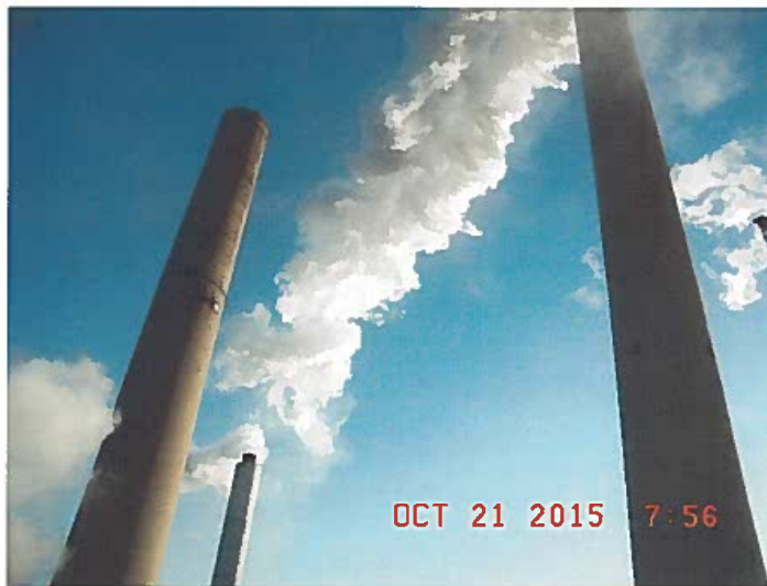
Stacks at Mill Creek Generating Station
