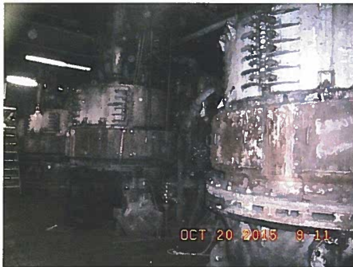
Unit 1 Pulverizers at Brown Generating Station
