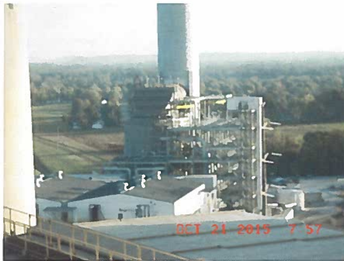
Unit 1 Scrubber at Mill Creek Generating Station
