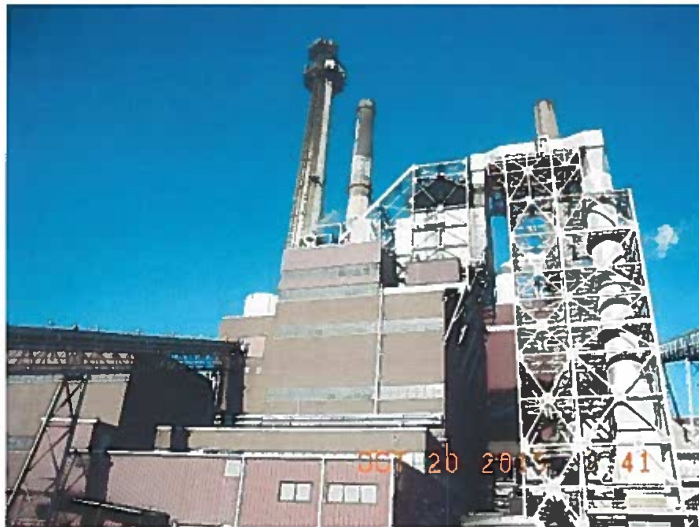
Units 1 & 2 at Brown Generating Station
