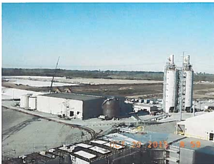
CCRT Building and Flyash Silos at Brown Generating Station
