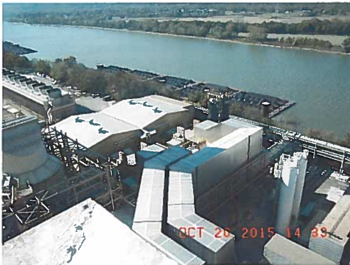
Unit 4 Baghouse at Ghent Generating Station
