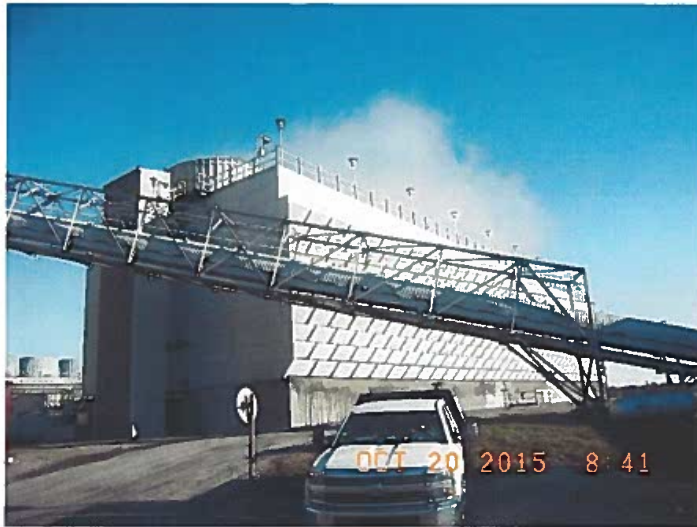
New Unit 1 Cooling Tower at Brown Generating Station
