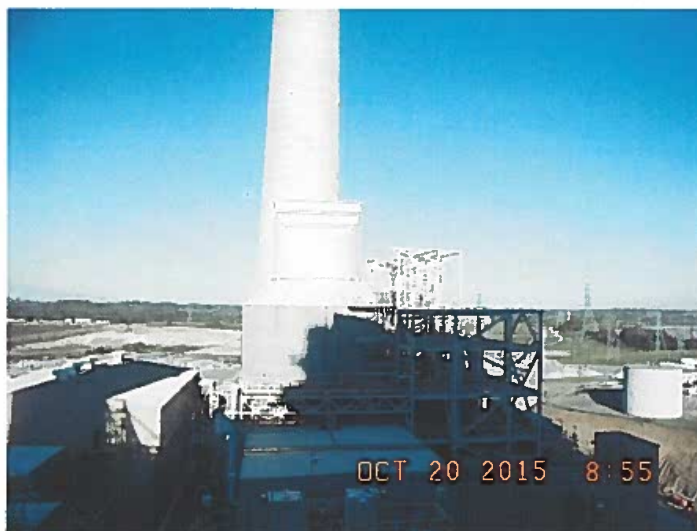
Scrubber at Brown Generating Station
