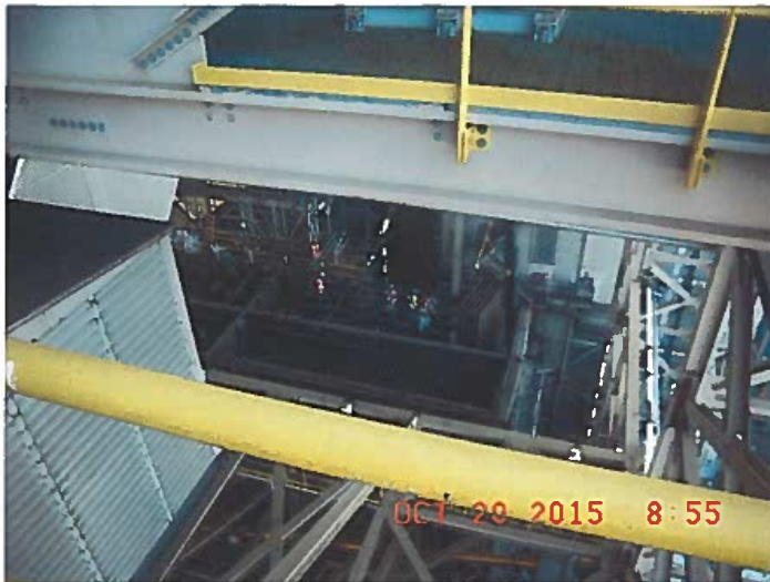
Precipitator (being demolished) at Brown Generating Station
