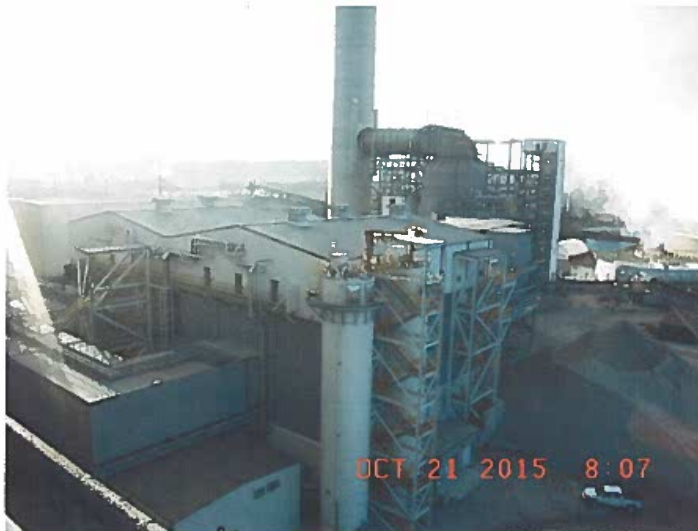
Unit 4 Scrubber at Mill Creek Generating Station
