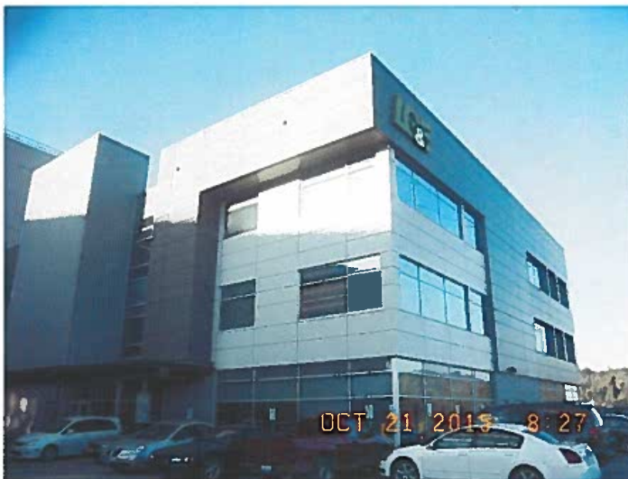
Administration Building at Mill Creek Generating Station
