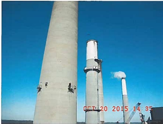
Units 1-3 Stacks at Ghent Generating Station
