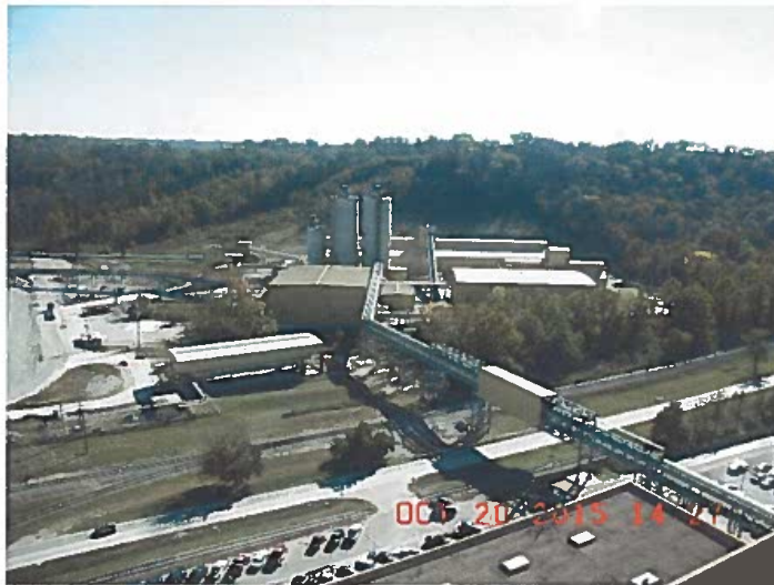
CCRT facility at Ghent Generating Station
