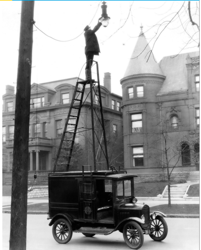
Concerns about lifetime and maintenance have been around for a long time. Credit: Ford Motor Company
