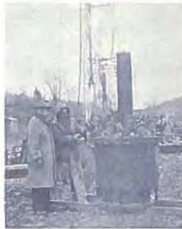
Milton J. Pfeiffer, CG & E vice-president, left, and Dale Erwin, Moran Brothers rig superintendent, inspect the 54-inch cutting tool.
