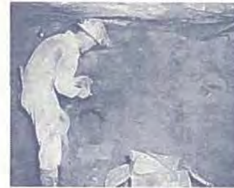
Workman loading dynamite in face of drift prior to blasting.
