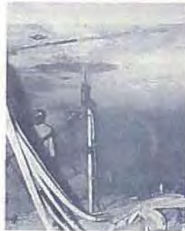
Installing roof bolts by means of air percussion hammer equipped with air lift jack.
