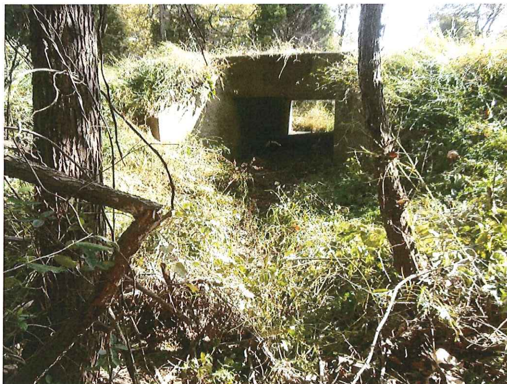
Photo 4: Little No Creek Looking Upstream from Stream Bed
