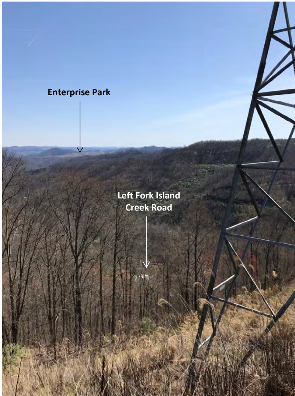
Photo 3. Facing southeast towards Enterprise Park from the Big Sandy – Broadford 765 kV Transmission Line
