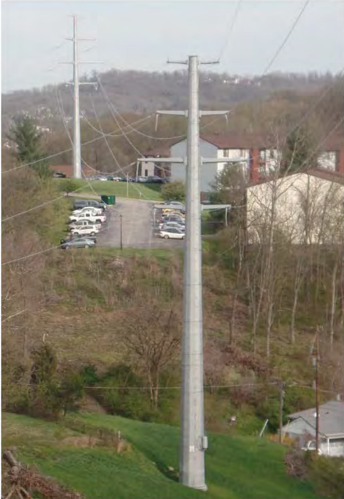
COMPARABLE STRUCTURE PHOTOGRAPH
