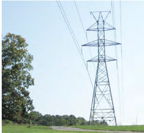
Figure 2. Proposed Typical Structure (Steel Lattice Tower)
