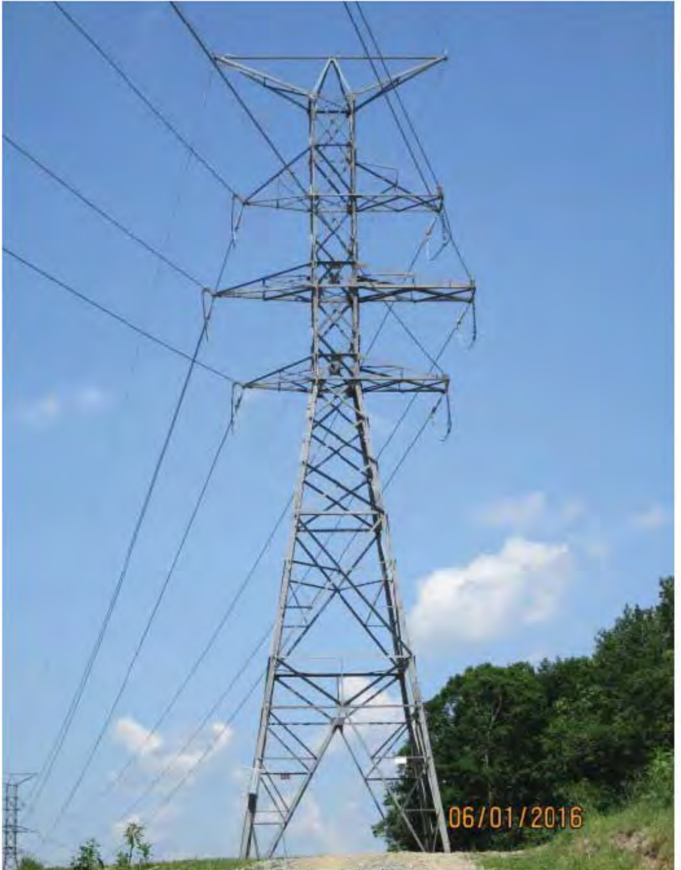
COMPARABLE STRUCTURE PHOTOGRAPH
