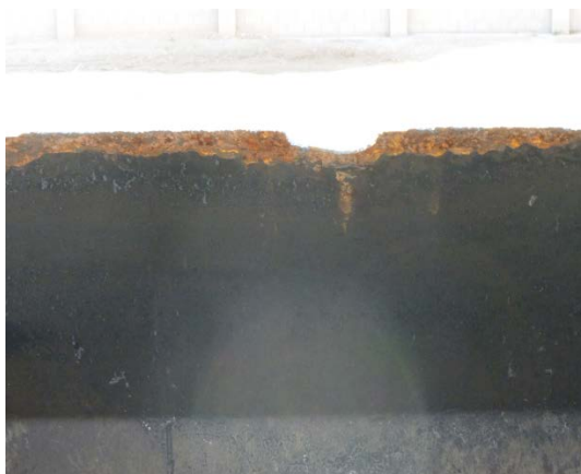
Corrosion of metal at wastewater treatment plants caused by H 2 S in covered basins. Plant about 8 years old.
