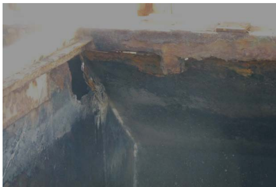
Corrosion of metal at wastewater treatment plants caused by H 2 S in covered basins. Plant about 8 years old.
