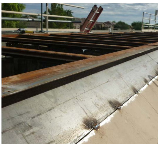
Repair of wastewater treatment tank replaced. Corroded metal removed for replacement
