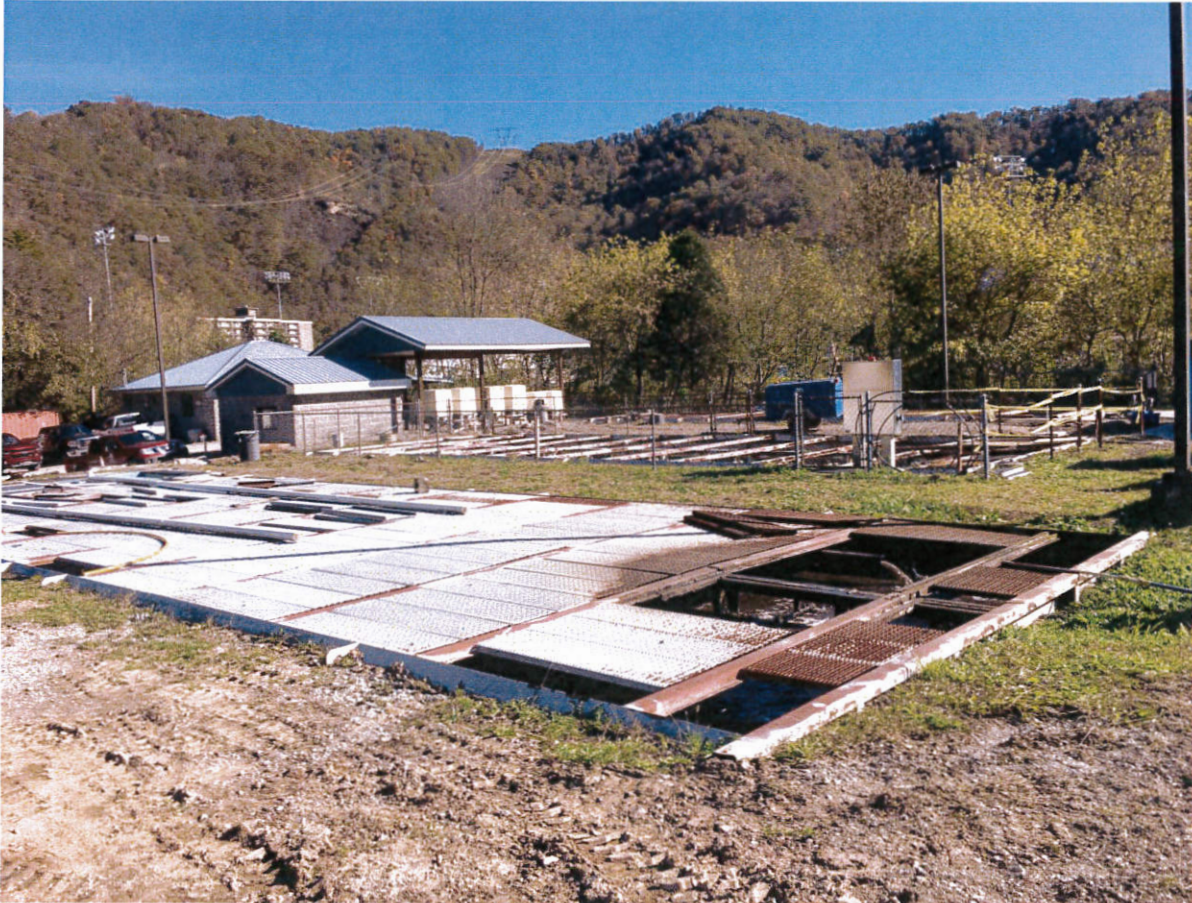
Douglas WWTP – Plant # 1 is still operational.
