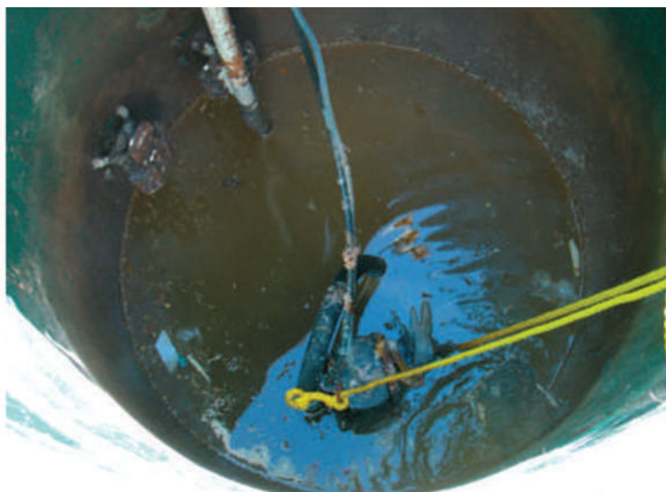
Top view showing Upgrade retrofit.
