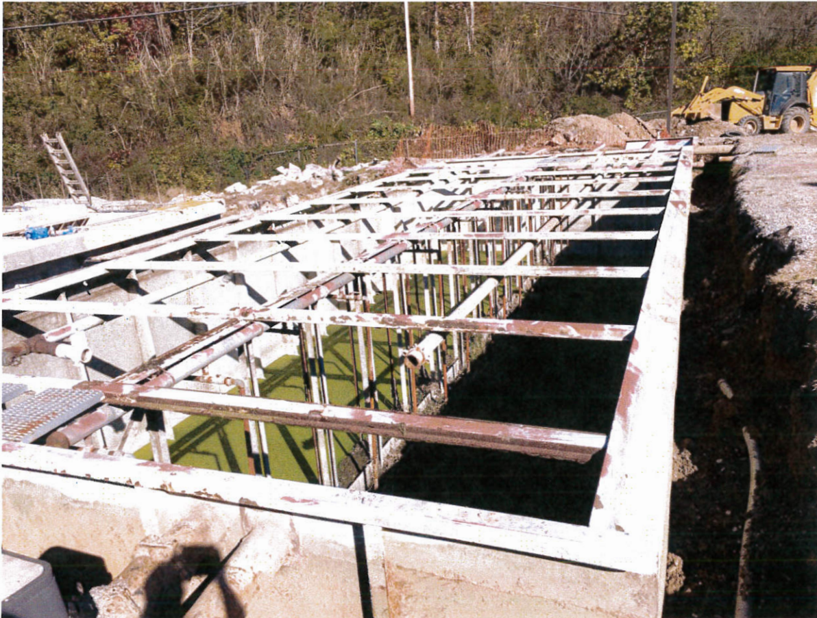
Douglas WWTP – Plant #2 has been taken out of service.
