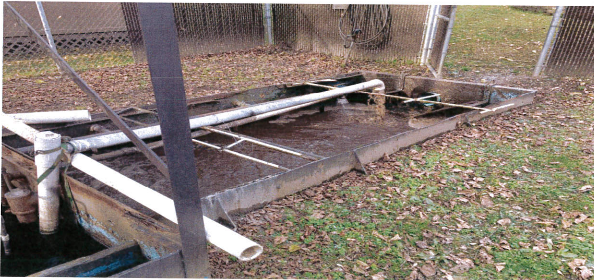
Maple Valley WWTP – Aeration Basin
