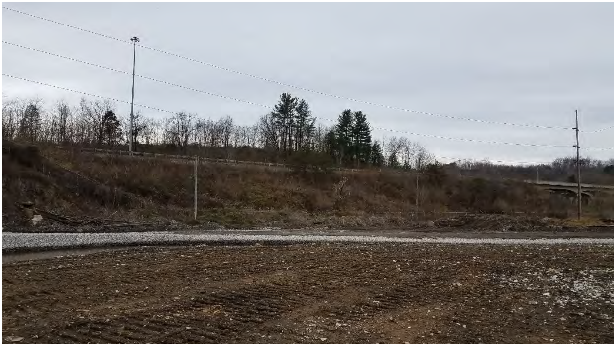
Photograph 5. Kentucky Electric Steel (KES) facility showing the Chadwick-KES 138kV Transmission Line and Interstate 64
