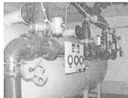
At no extra or hidden cost to the District, Alliance developed five-year plans for the water and sewer systems, as well as a five-year financial plan.
