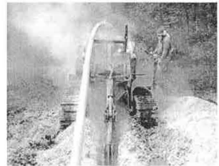
Savings from an Alliance-assisted water-loss reduction project was more than $70,000 in one year.
