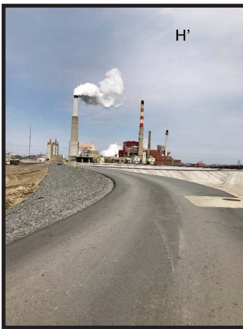
Photo H': Road along Sediment/Stormwater Pond 1
