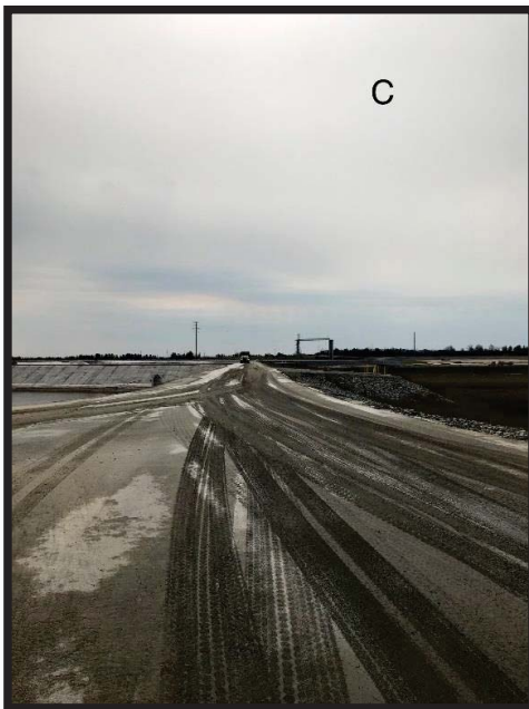
Photo C: Road along Sediment/Stormwater Pond 2
