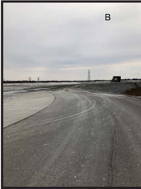
Photo B: Road along Coal Combustion Residual Treatment Material Handling Area
