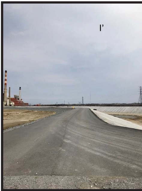
Photo I': Road along Sediment/Stormwater Pond 1
