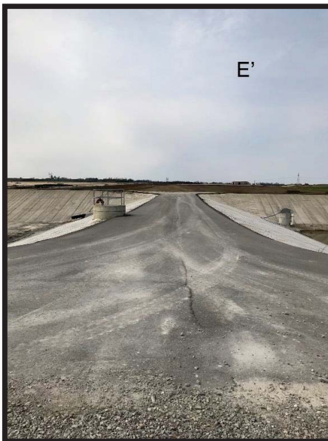
Photo E': Road between Sediment/Stormwater Pond 2 and Leachate Pond Area
