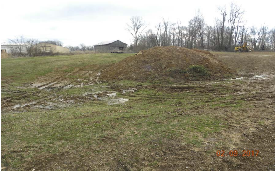
View of the Project Site from the northwest property corner and the area of Boring No. 1
