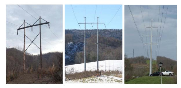
Figure 1: Existing (left), Proposed Steel H-Frame (middle), and Proposed Double Circuit Monopole (right)
