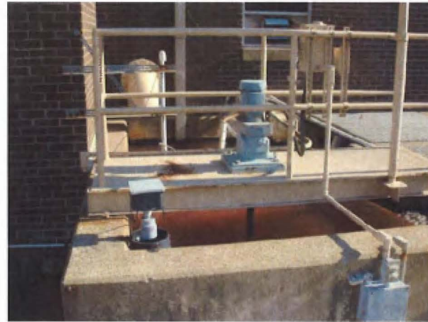
Figure 5.02-1 Existing Rapid Mix Basin
