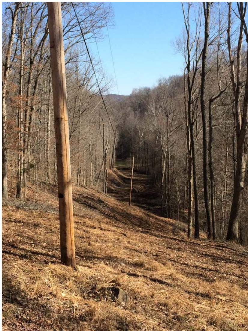
Completed Task 2 work on Greysbranch - Greysbranch Circuit in Greenup County
