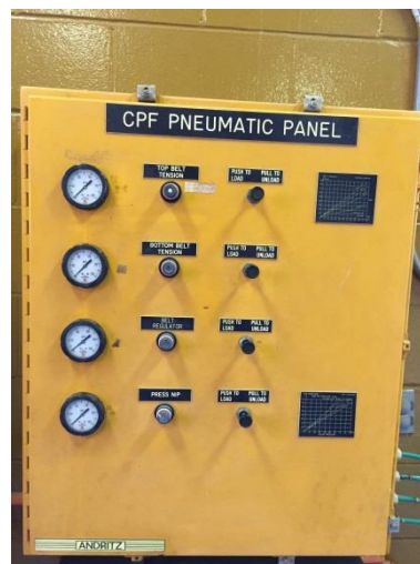
Figure 10 – Pneumatic Control Panel Assembly
