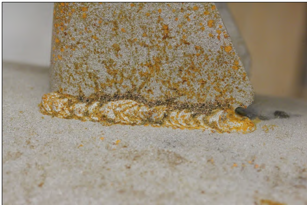
Figure 9. Image of the Lug B4 exterior weld which exhibited substantial fusion except for undercut and arc strikes.
