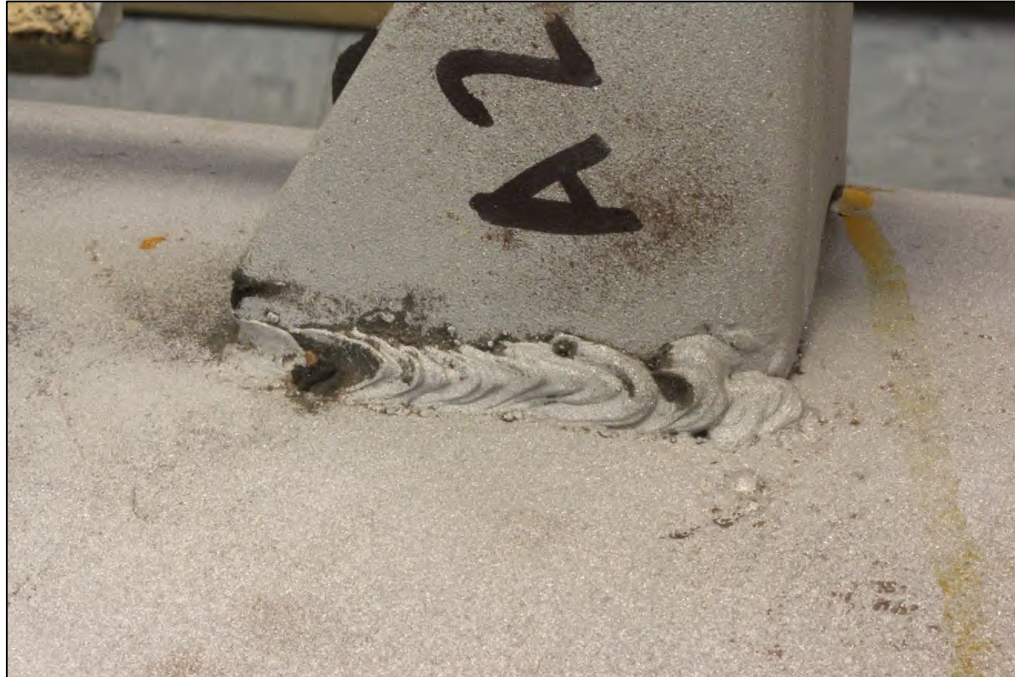
Figure 6. Image of the Lug A2 exterior bottom weld which exhibited substantial fusion except for some undercut, spatter, and arc strikes.
