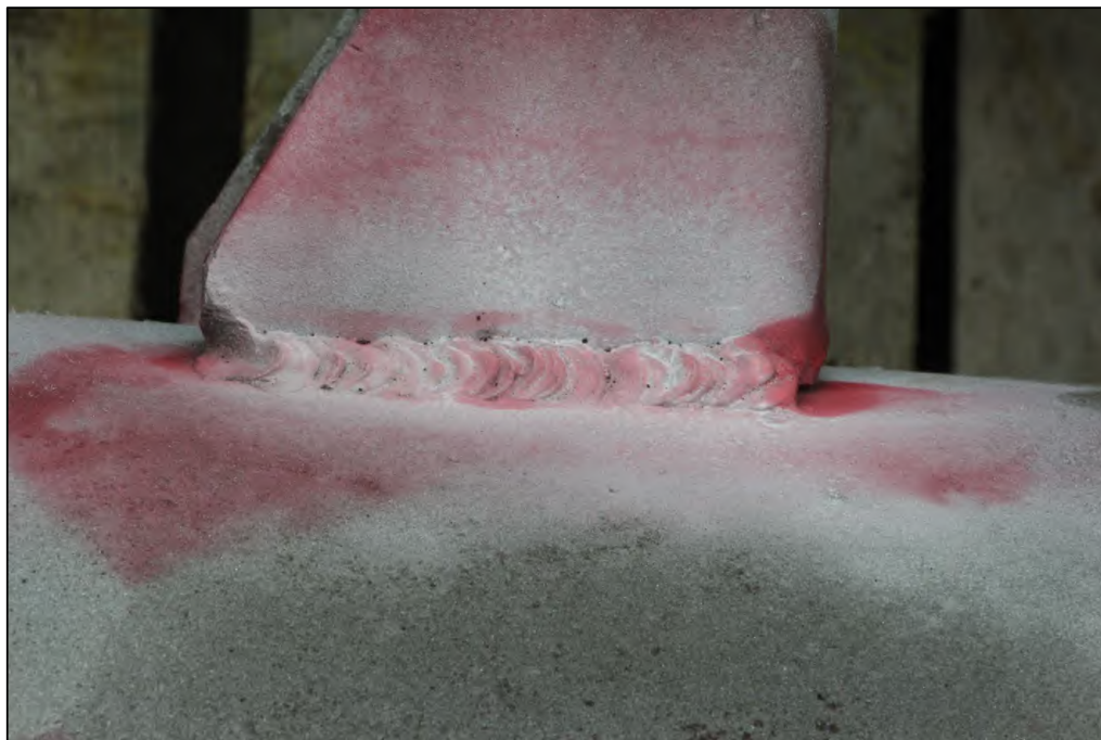
Figure 12. Image of the Lug B1 exterior top weld after dye penetrant media had been used during inspection.
