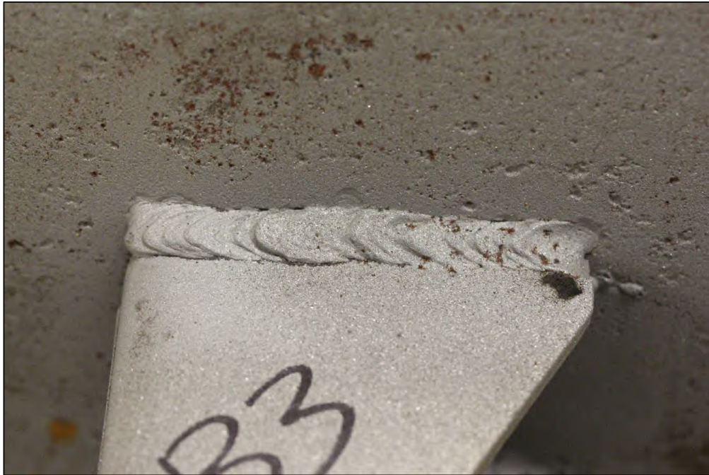
Figure 9. Image of the Lug B3 weld which exhibited substantial fusion except for some undercut and spatter.
