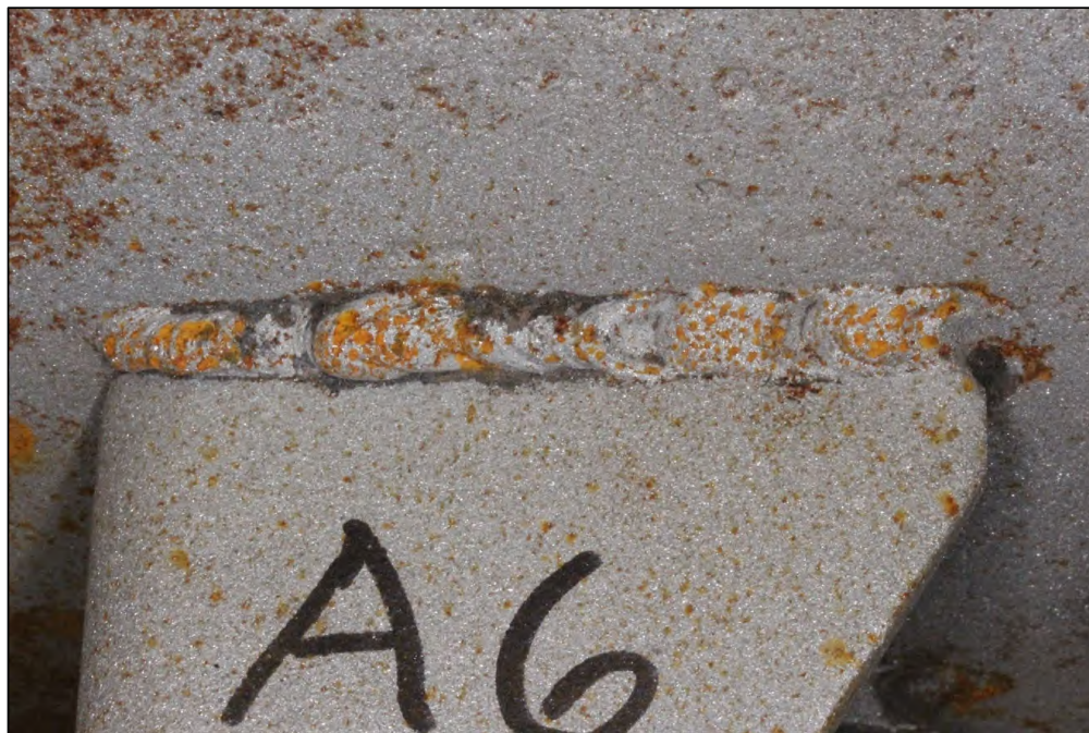
Figure 7. Image of the Lug A6 exterior bottom weld which exhibited substantial fusion except for some undercut regions.
