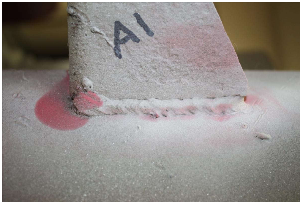
Figure 9. Image of the Lug A4 exterior top weld after dye penetrant media had been used during inspection.
