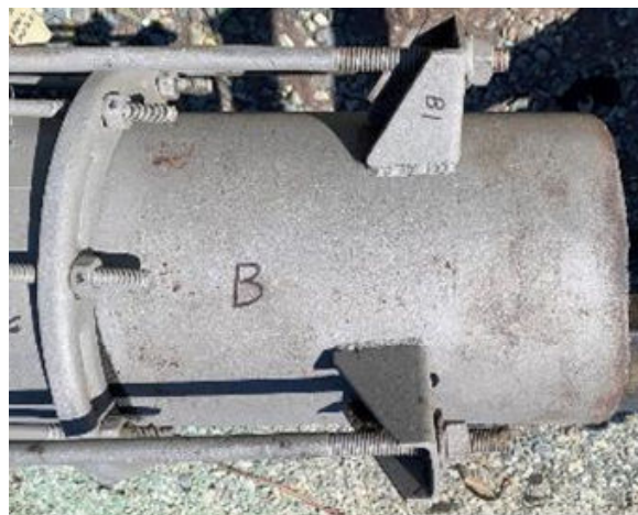
Figure 3 – Pipe Side B
