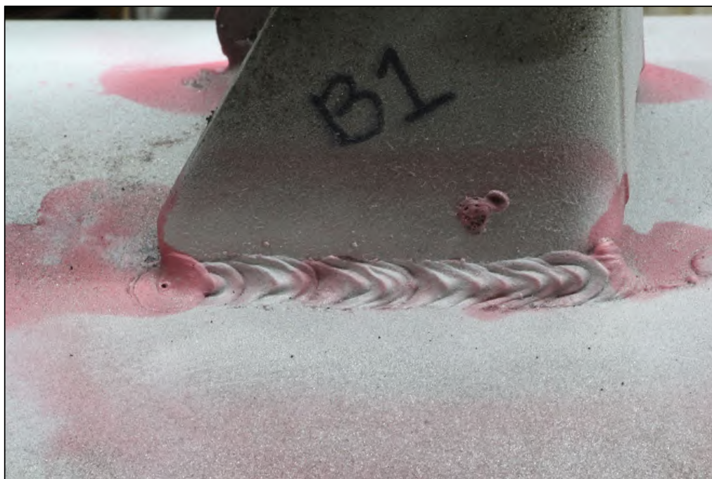
Figure 11. Image of the Lug B1 exterior top weld after dye penetrant media had been used during inspection.
