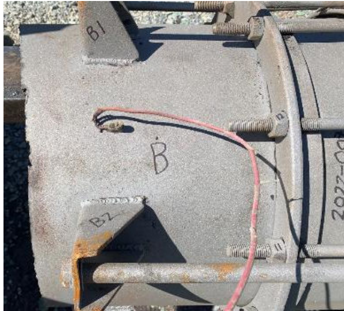
Figure 3 – Pipe Side B
