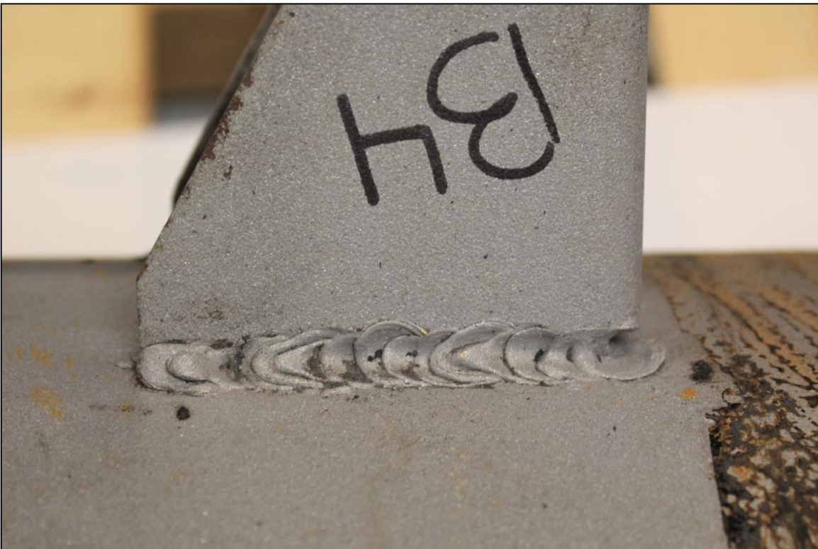
Figure 10. Image of the Lug B4 exterior bottom weld which exhibited substantial fusion except for undercut, and porosity.
