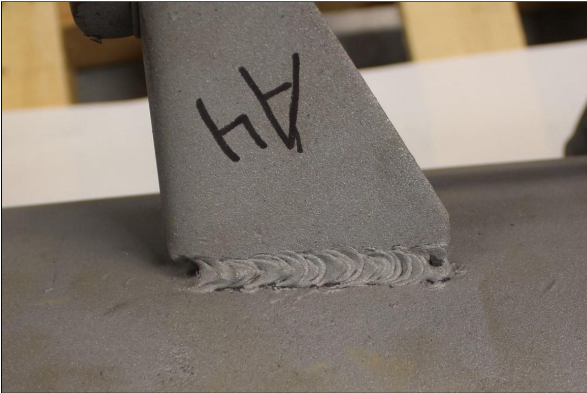
Figure 7. Image of the Lug A4 exterior bottom weld which exhibited substantial fusion except for some undercut and porosity.
