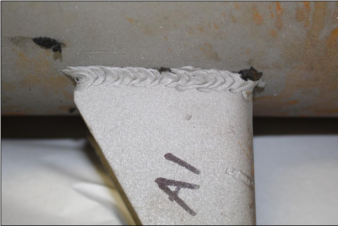
Figure 5. Image of the Lug A1 exterior bottom weld which exhibited substantial fusion except for some undercut, porosity, and arc strikes.
