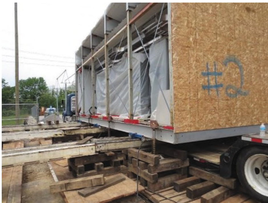
Figure 27: Modular control house being delivered.
