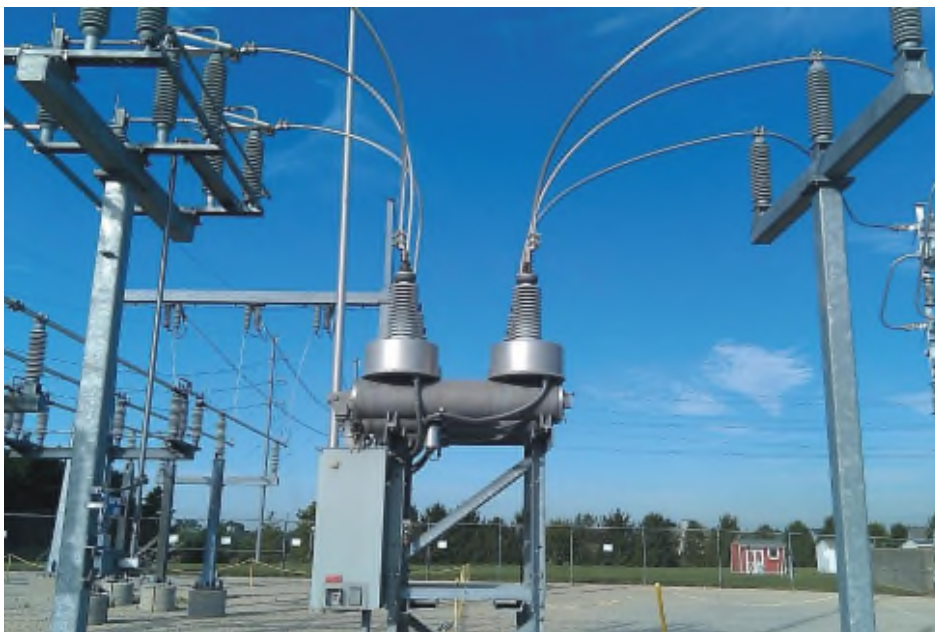
Figure 21: New circuit breaker installation inside the substation.
