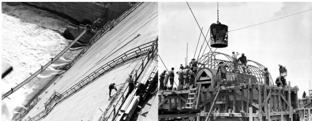
TVA pretty much invented utility economic development. Here workers are shown in the 1930s constructing the Norris Dam, TVA's first hydroelectric project, where the agency this summer commemorated the dam's 80th anniversary of operations.
