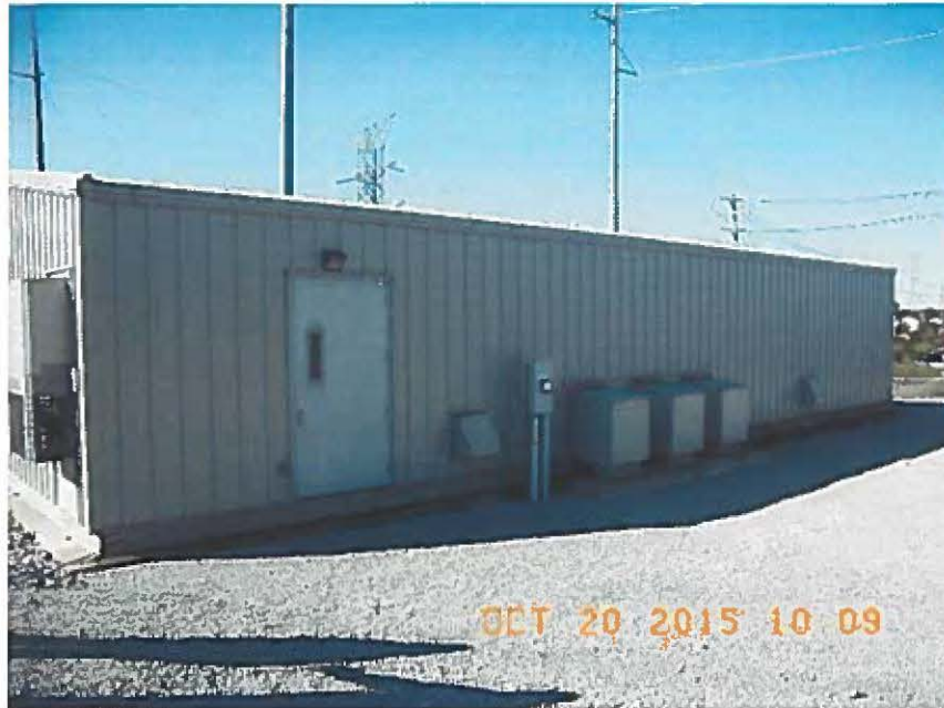
Control Building at Higby Mill Substation
