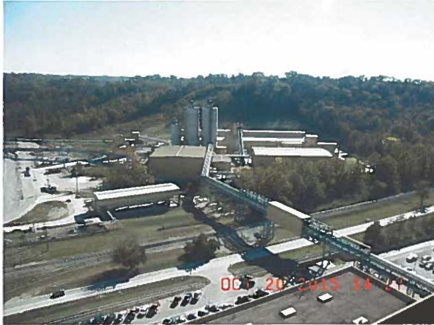
CCRT facility at Ghent Generating Station
