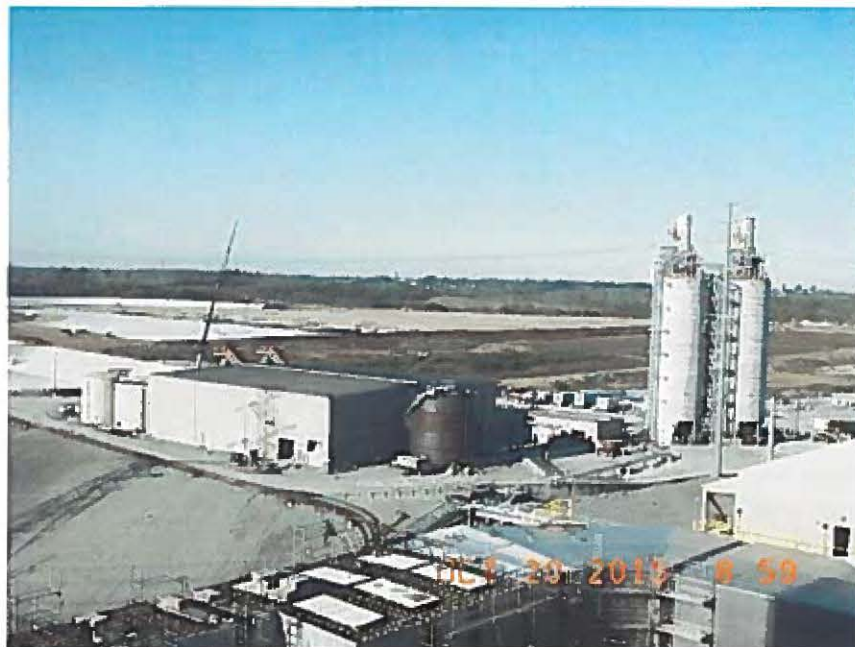
CCRT Building and Flyash Silos at Brown Generating Station
