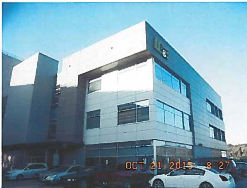
Administration Building at Mill Creek Generating Station
