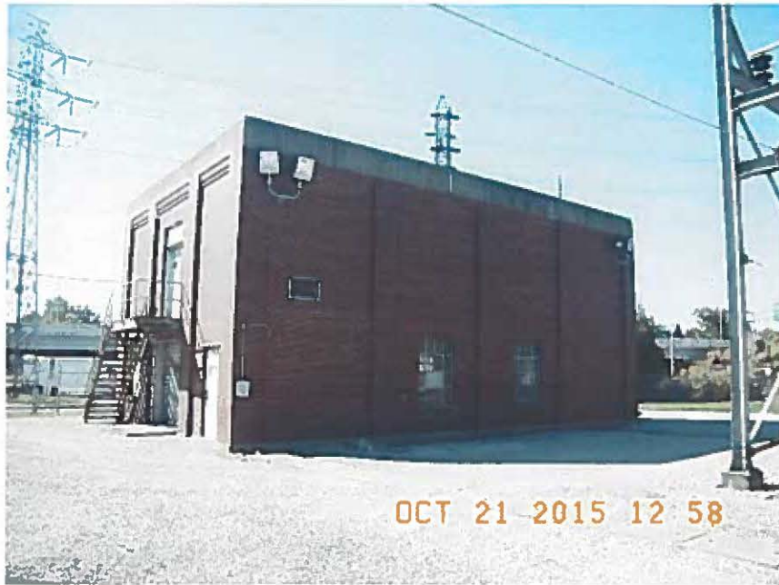
Control Building at Canal Substation
