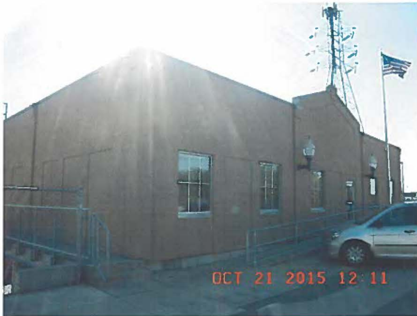
New Administration Building at Ohio Falls Hydro Plant
