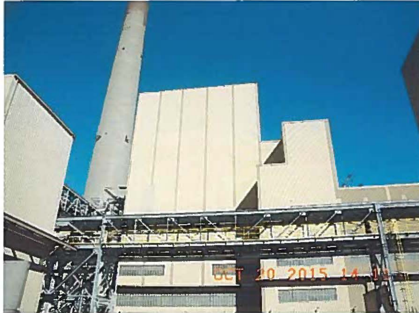
Unit 4 Boiler at Ghent Generating Station
