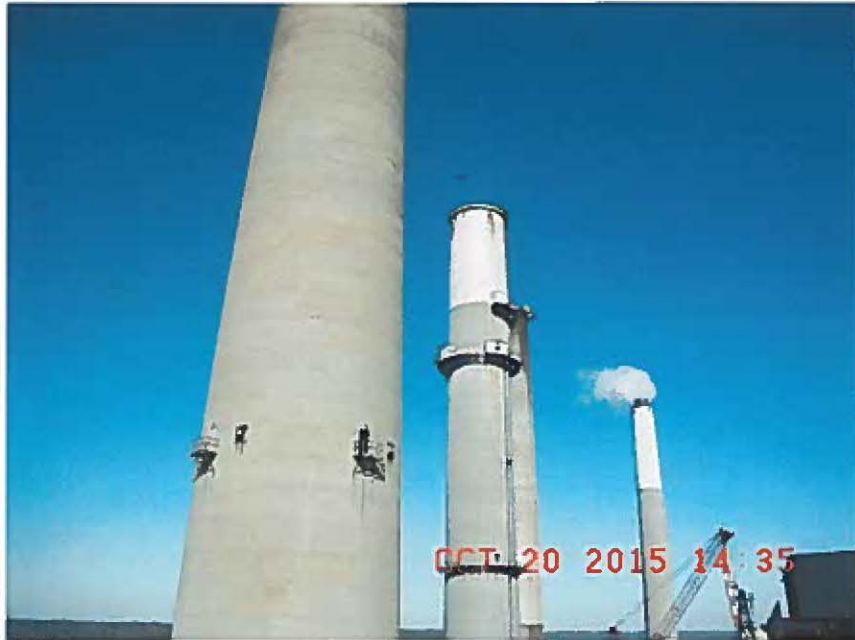
Units 1-3 Stacks at Ghent Generating Station
