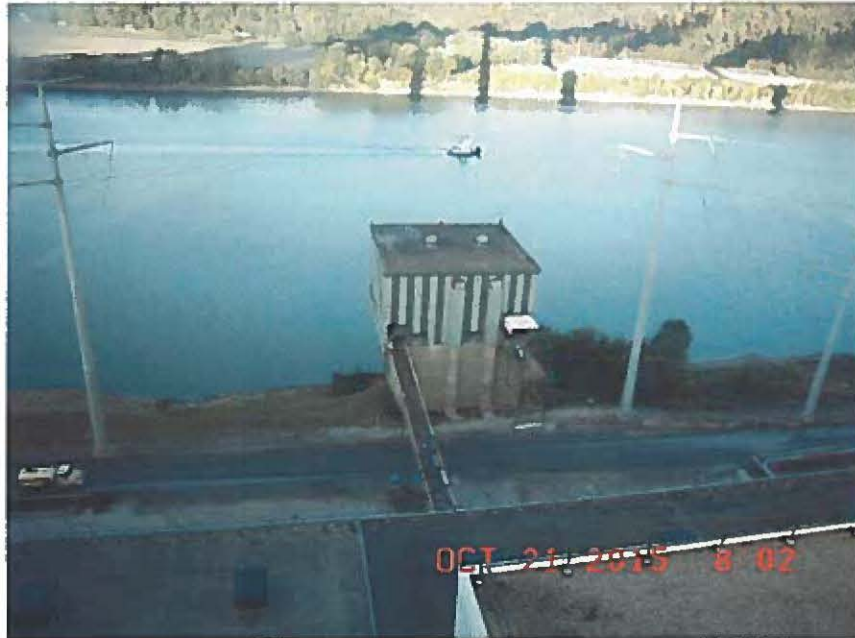
Intake at Mill Creek Generating Station
