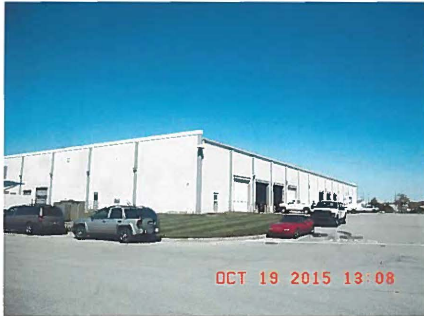
Garage at Auburndale Service Center
