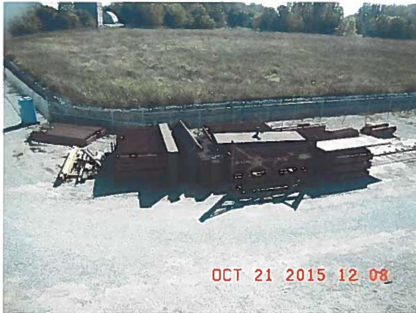
Trash Racks (soon to be installed) at Ohio Falls Hydro Station
