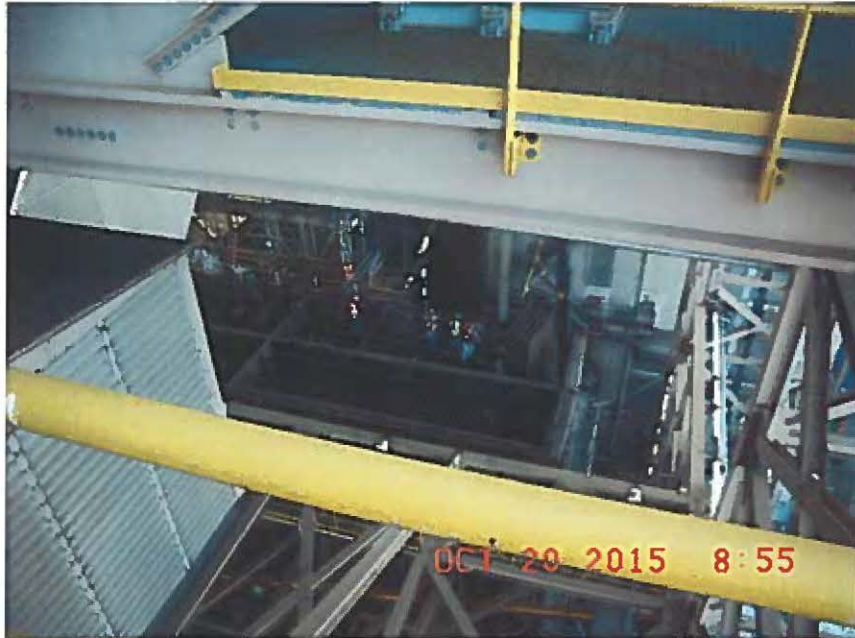
Precipitator (being demolished) at Brown Generating Station
