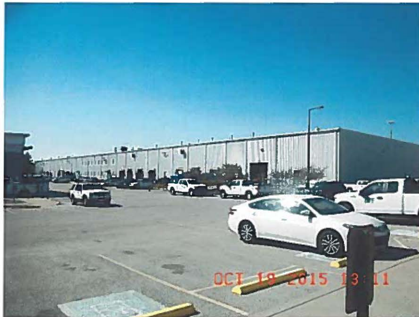
Warehouse at Auburndale Service Center
