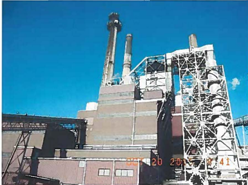
Units 1 & 2 at Brown Generating Station
