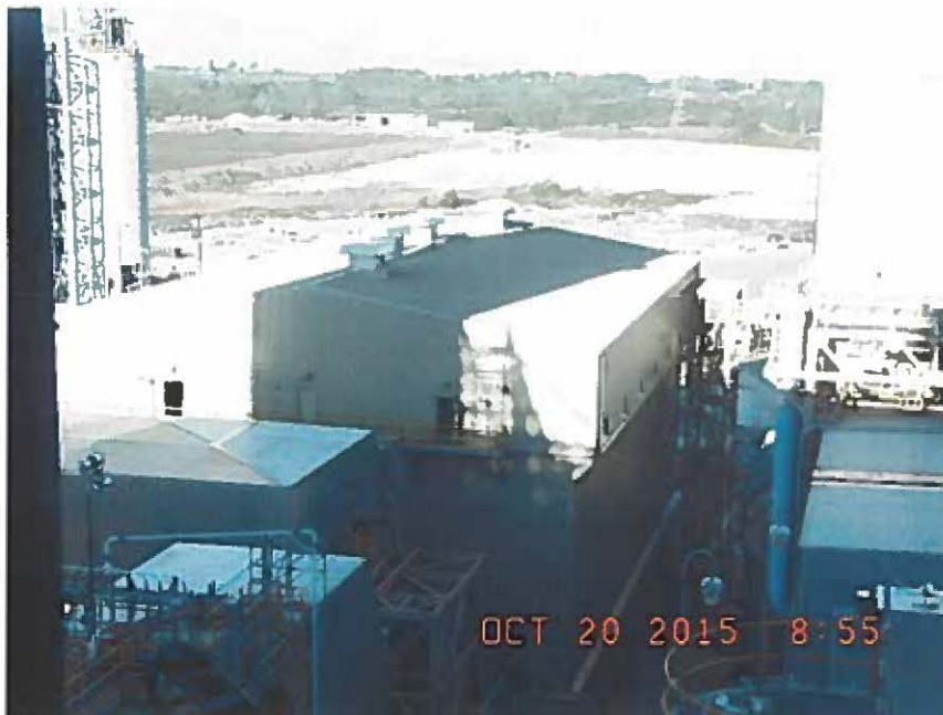
Baghouse at Brown Generating Station
