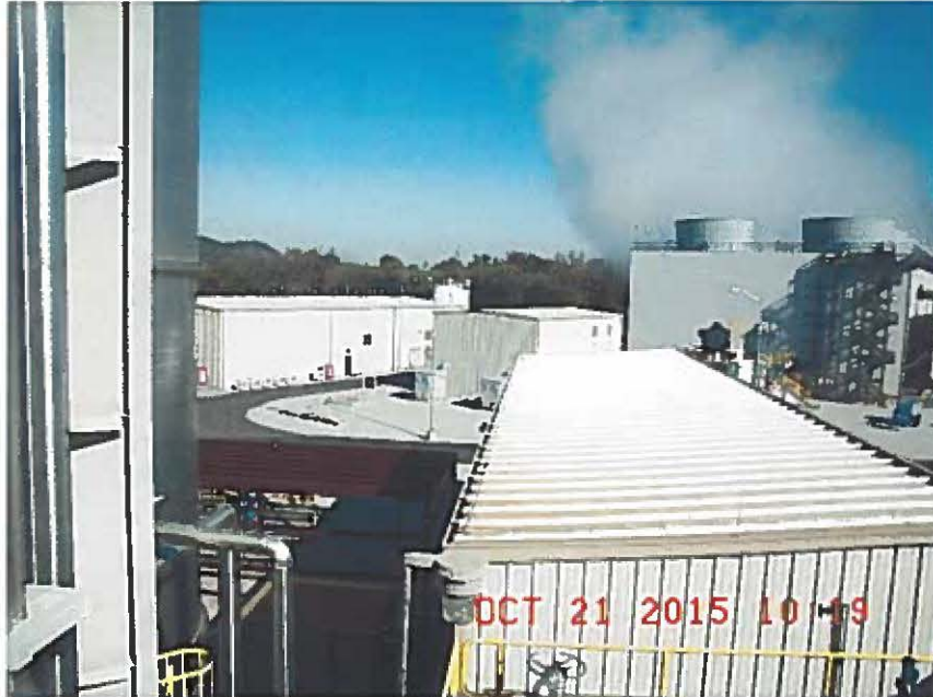
Gas Compressor and Water Treatment Buildings at Cane Run Unit 7
