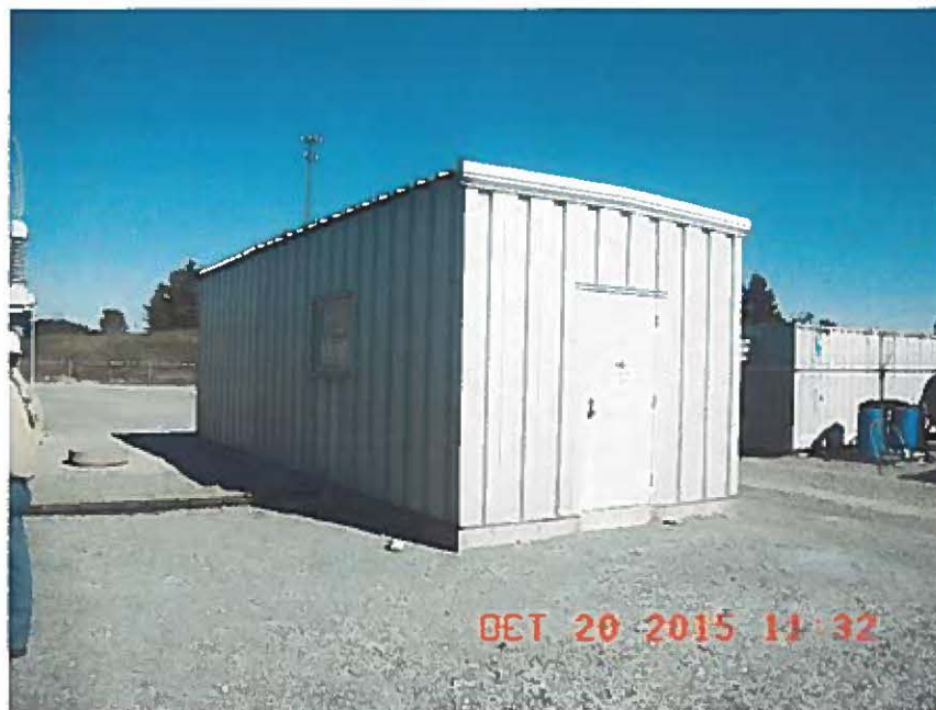
Control Building at Toyota North Substation
