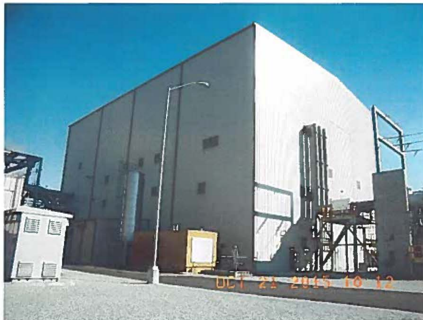
Steam Turbine Building at Cane Run Unit 7
