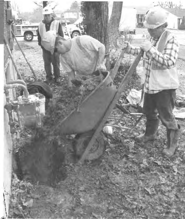
The service riser is a piping component of the natural gas service line that protects the plastic gas service pipe as it transitions from below ground to above ground and from plastic to steel just upstream of LG&E's gas meter.
