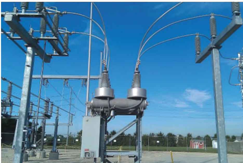
Figure 21: New circuit breaker installation inside the substation.
