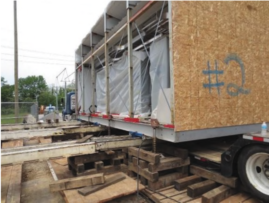
Figure 27: Modular control house being delivered.
