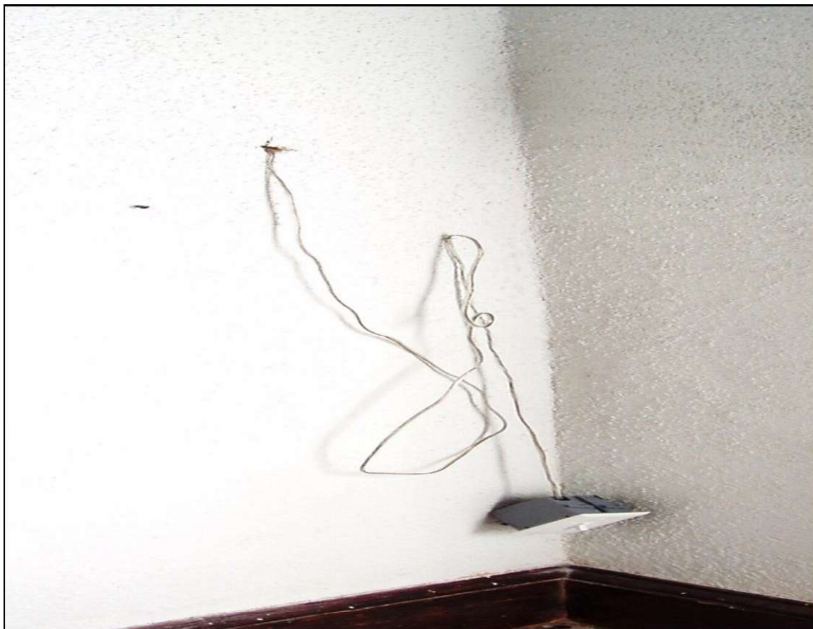
Figure 4-9 Toggle switch controlling the meter bypass
