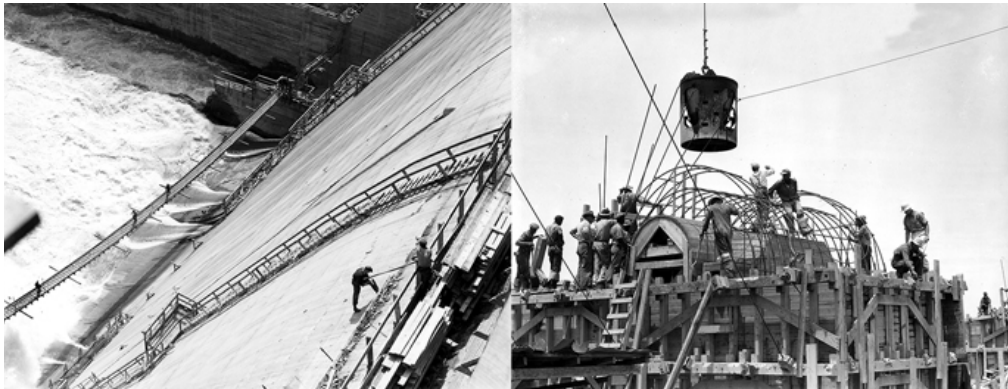
TVA pretty much invented utility economic development. Here workers are shown in the 1930s constructing the Norris Dam, TVA's first hydroelectric project, where the agency this summer commemorated the dam's 80th anniversary of operations.
