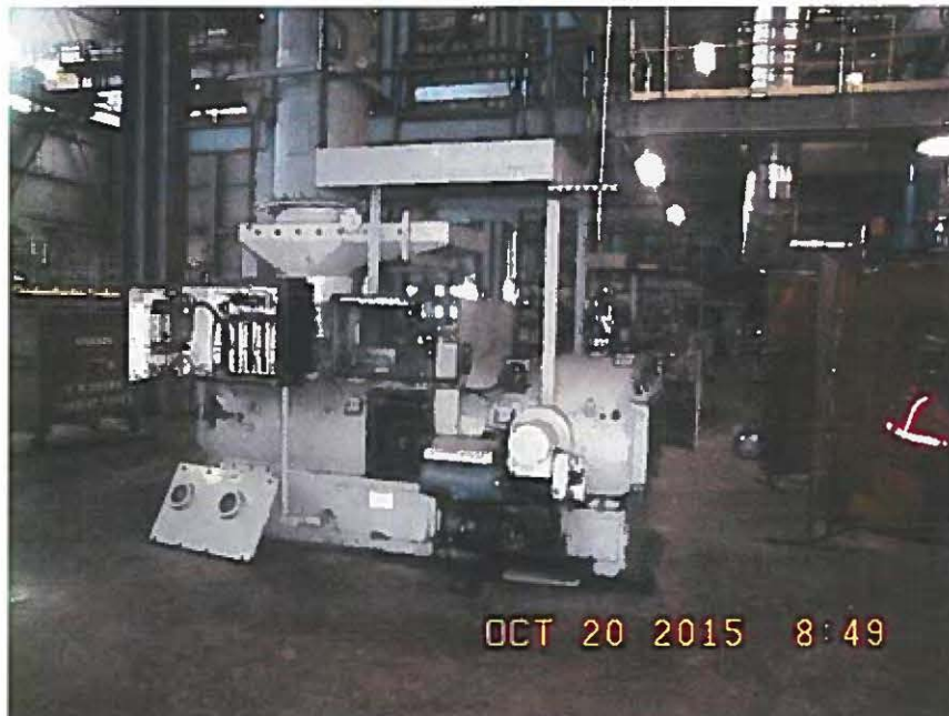
Unit 3 Coal Feeders at Brown Generating Station
