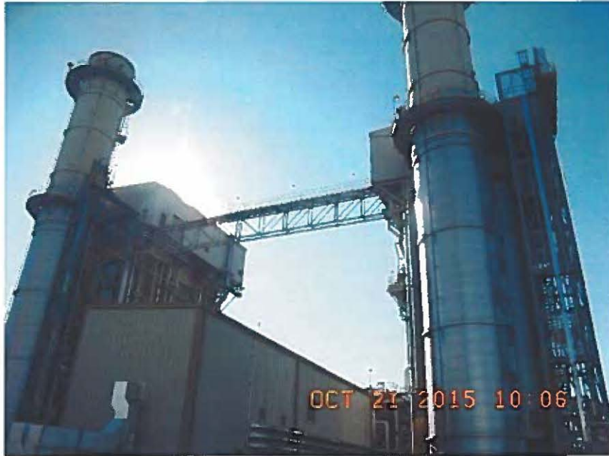
HRSGs at Cane Run Unit 7 Generating Station
