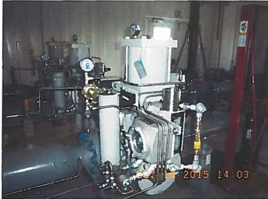
Regulator Runs at Penile City Gate Station
