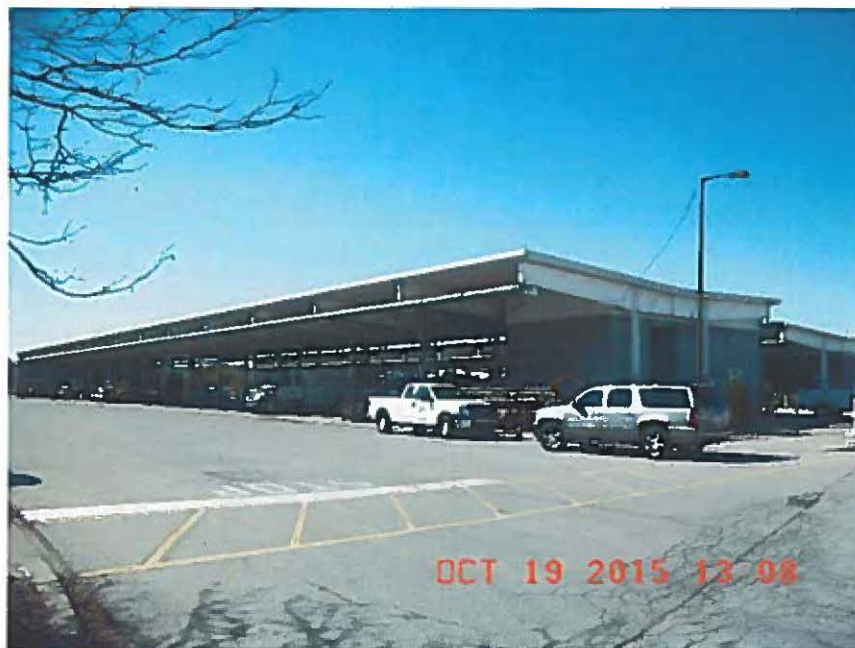
Vehicle Canopy at Auburndale Service Center
