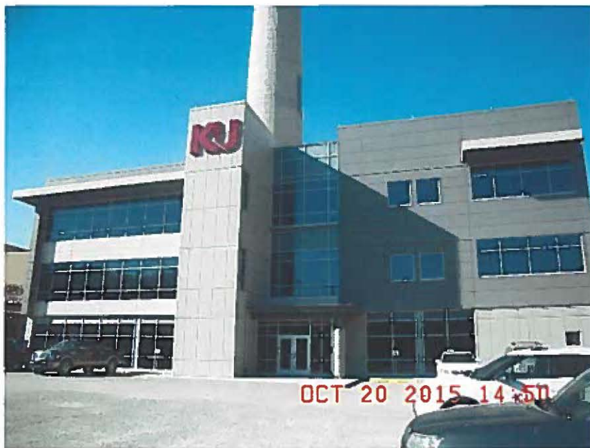
Administration Building at Ghent Generating Station
