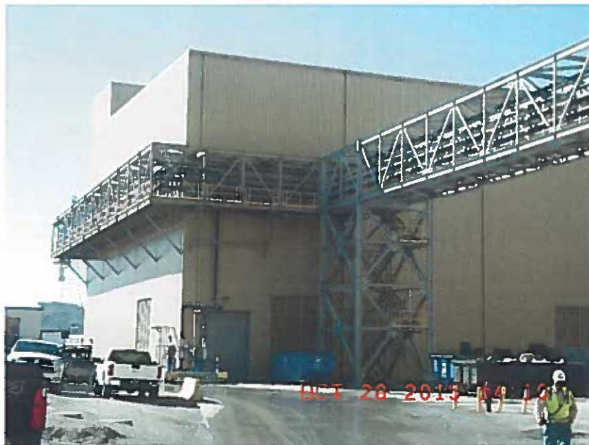
Limestone Prep Building at Ghent Generating Station
