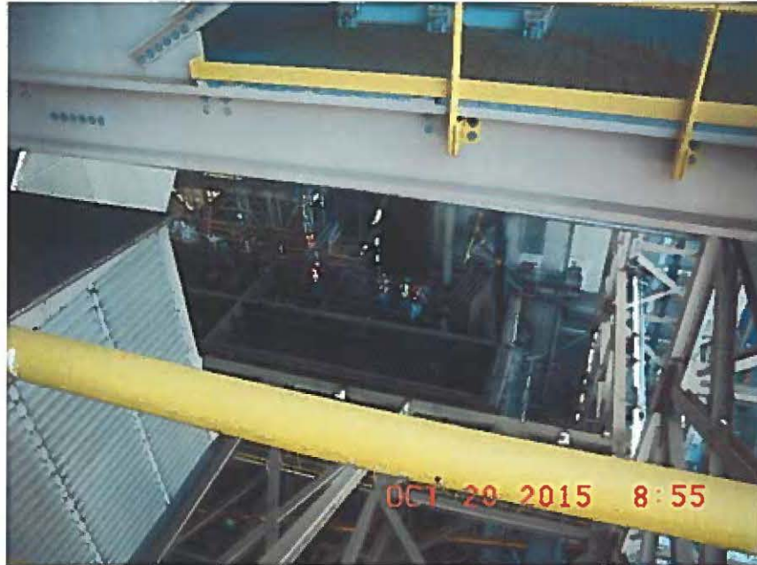
Precipitator (being demolished) at Brown Generating Station
