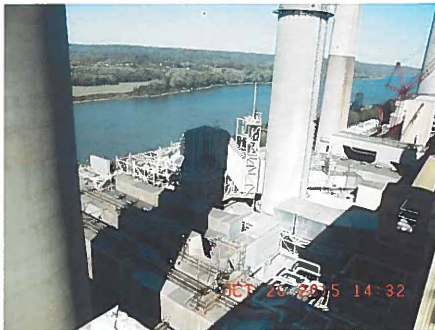
Unit 3 Scrubber at Ghent Generating Station
