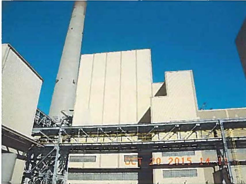
Unit 4 Boiler at Ghent Generating Station
