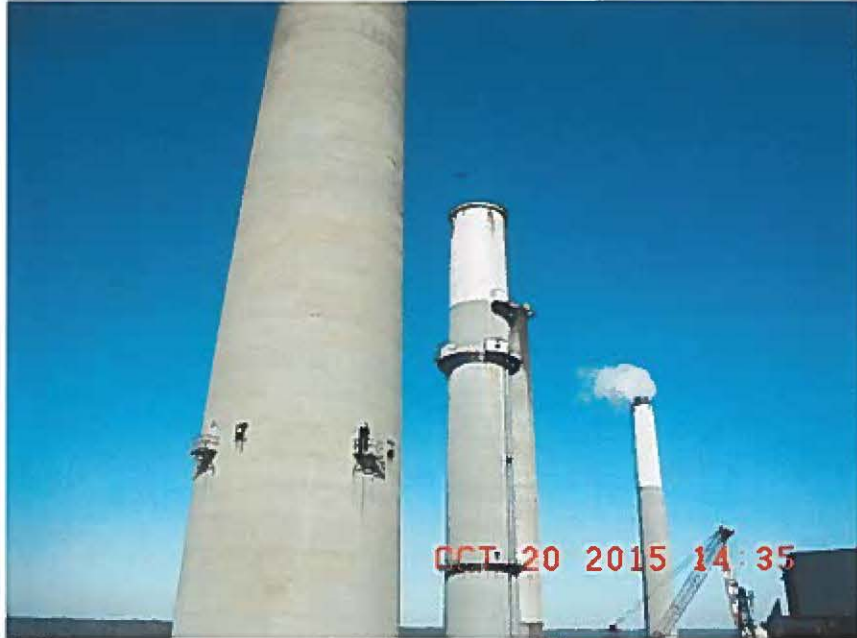
Units 1-3 Stacks at Ghent Generating Station
