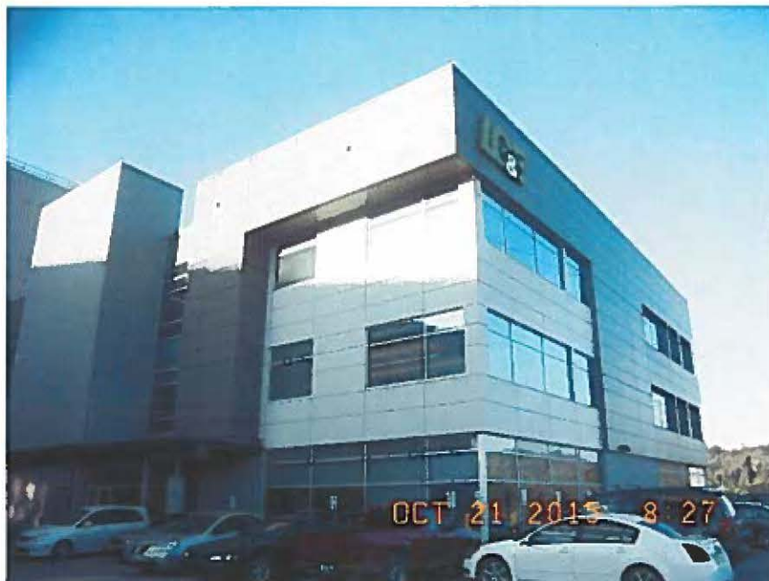
Administration Building at Mill Creek Generating Station
