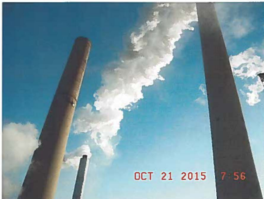
Stacks at Mill Creek Generating Station
