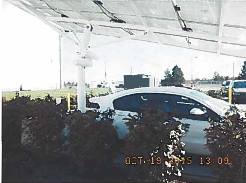
EU Charging Station at Auburndale Service Center
