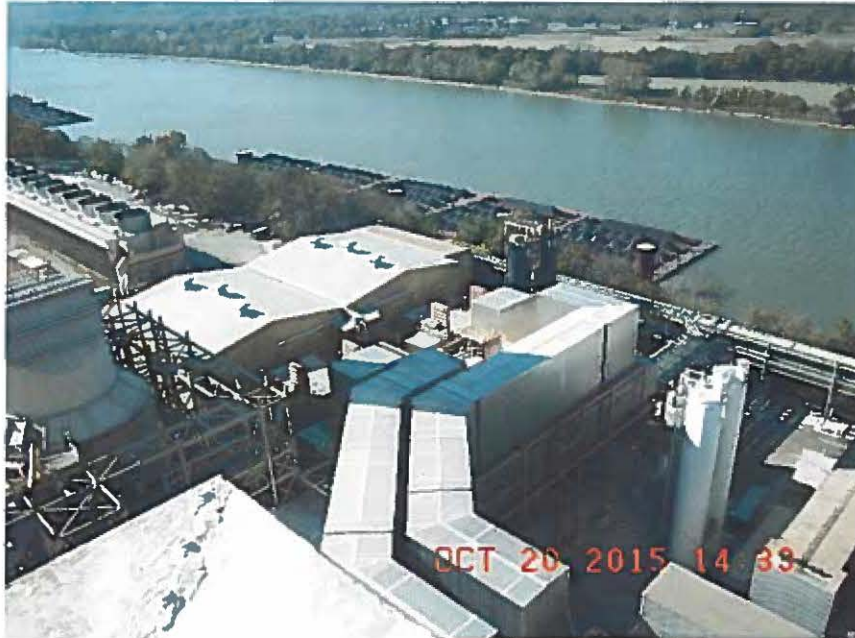
Unit 4 Baghouse at Ghent Generating Station
