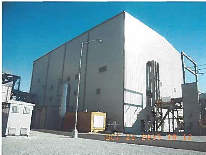
Steam Turbine Building at Cane Run Unit 7
