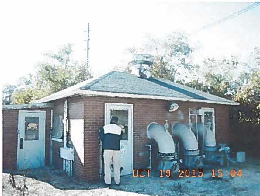
Regulator Building at St. Helens Regulator Station
