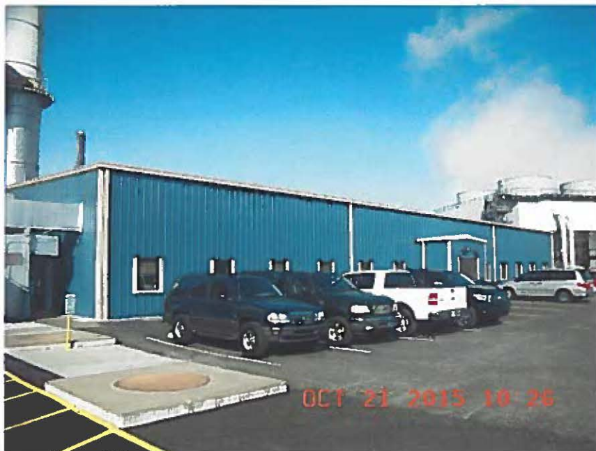
Office at Cane Run Unit 7 Generating Station
