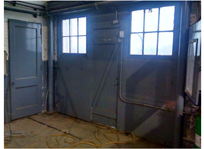
EXISTING DOOR, WINDOW, AND WALL FRAMING TO BE REMOVED
