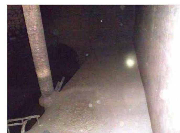
PLATFORM AT ELEV. 471 LOOKING WEST FROM LADDER
