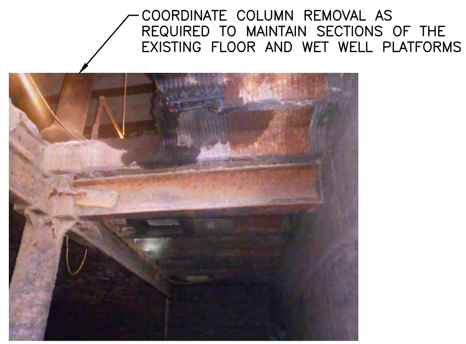
UNDERSIDE VIEW OF PLATFORM AT ELEV. 483.40
