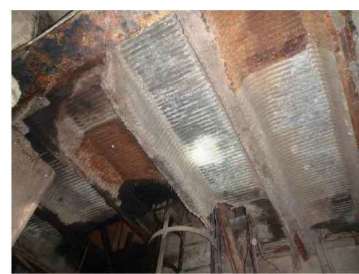
UNDERSIDE VIEW OF PLATFORM AT ELEV. 483.40
