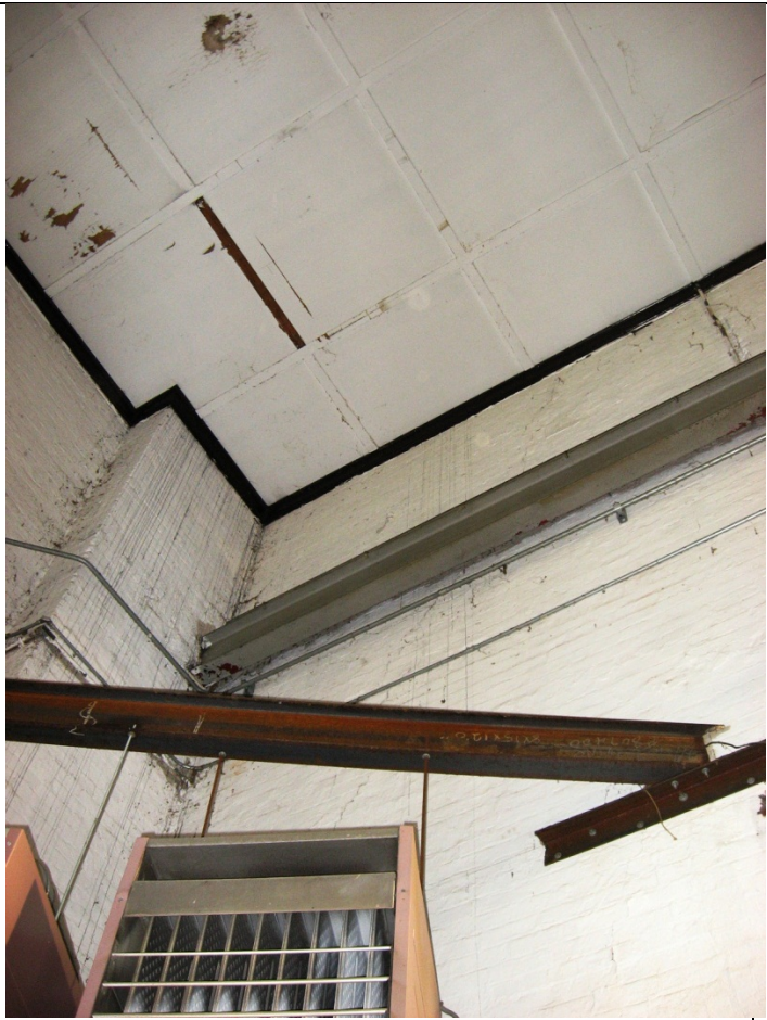
Ctr Wall Reflected Crack 85
