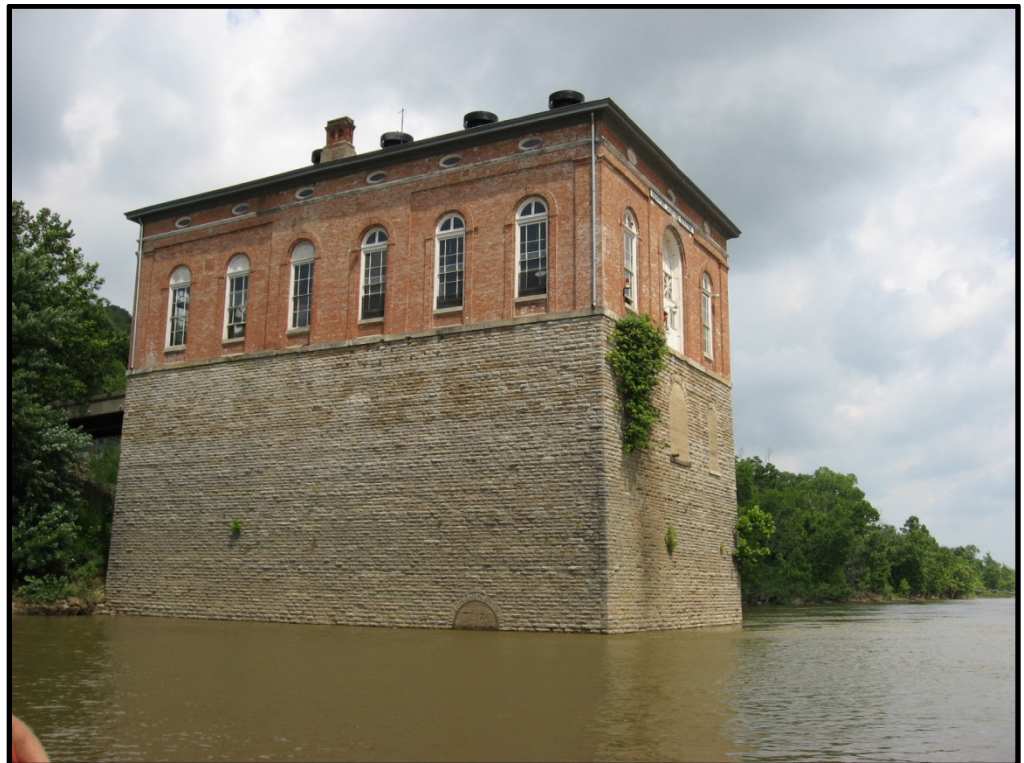
Photo 4.1: ORPS2 Facility Looking Downstream
