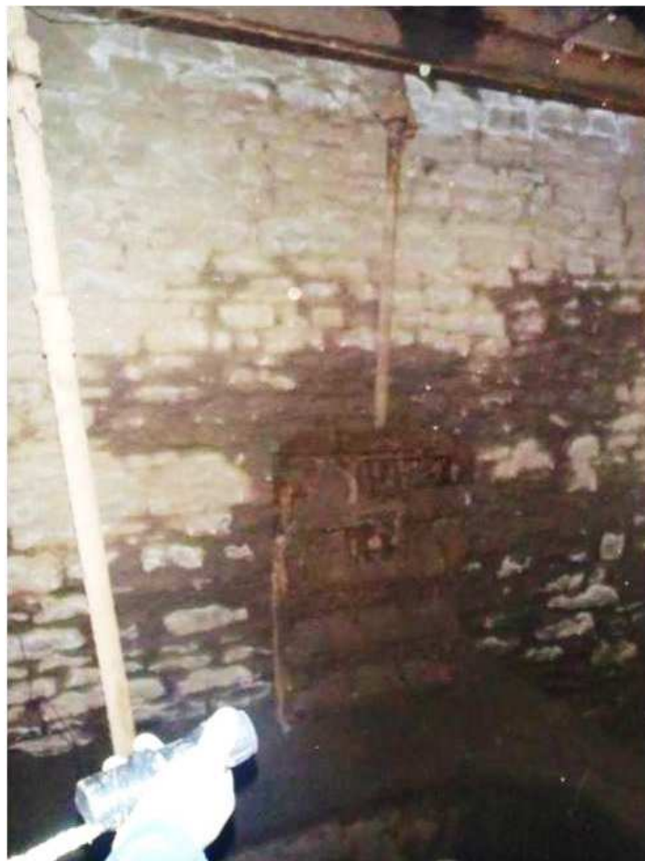
Figure 1 - Photo of existing sluice gate from dive inspection (photo by Marine Solutions Inc. (MSI))
