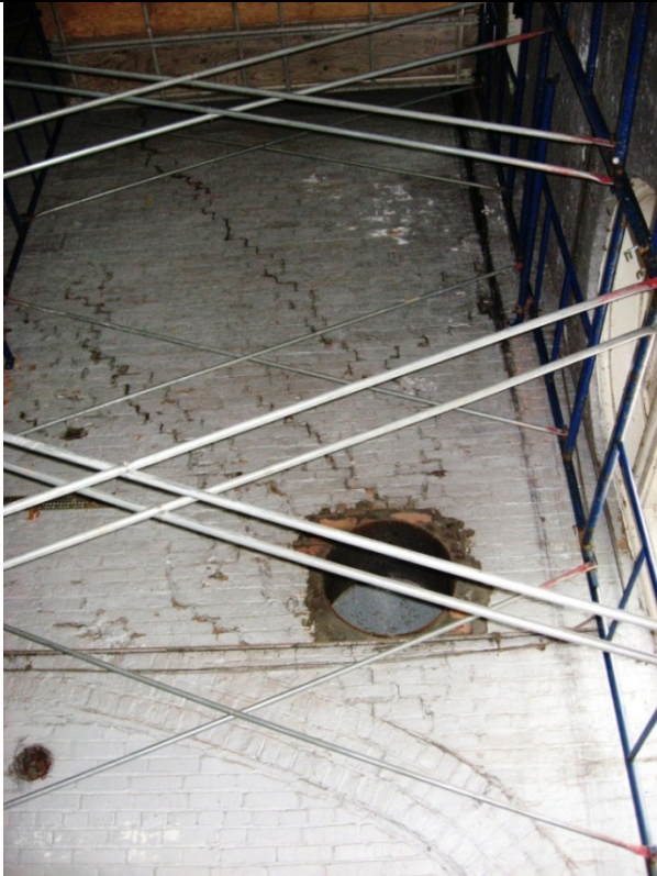
Center Wall South 86
