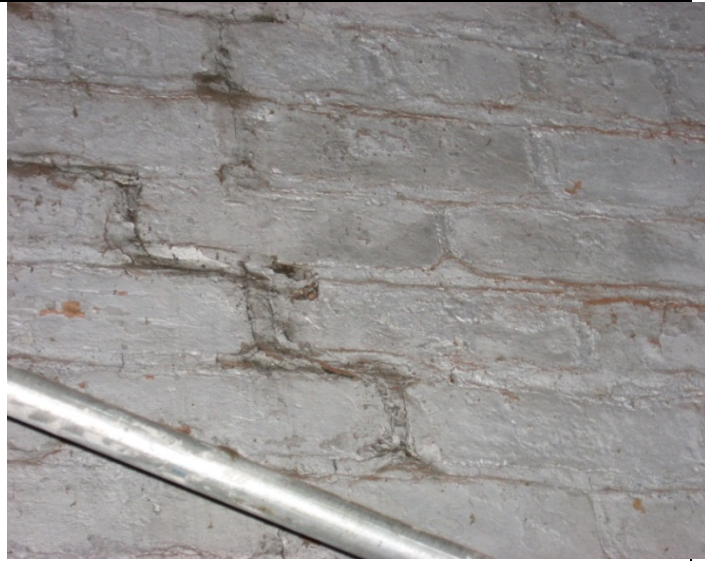
Inactive Crack 29
