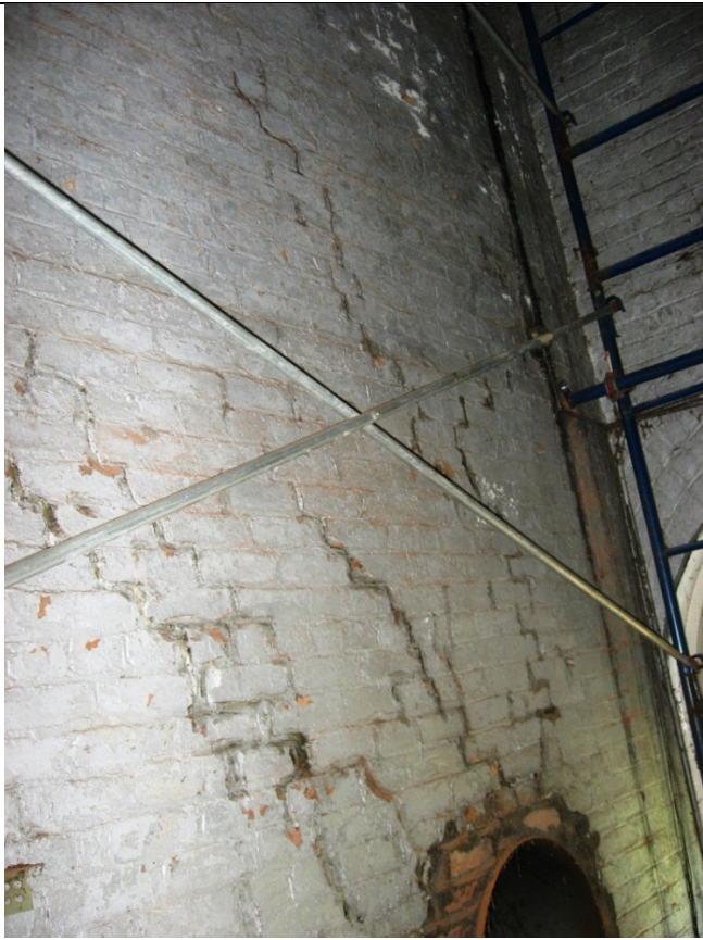
Center Wall South End 91
