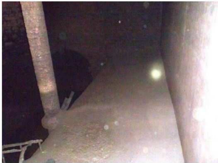
Figure 3 - Platform at Elevation 471.0 (Photo by MSI)
