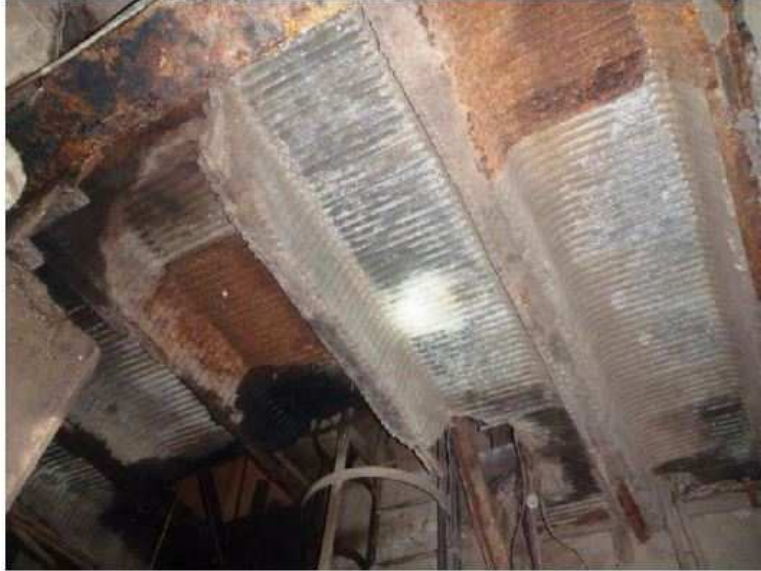
Figure 2 - Underside of platform at Elevation 483.4 (Photo by MSI)
