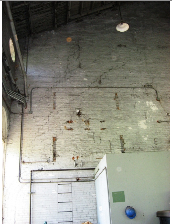
Center Wall South End Look West 04
