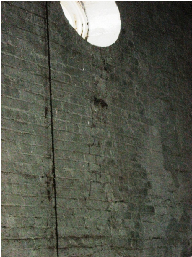
Inactive Crack 94
