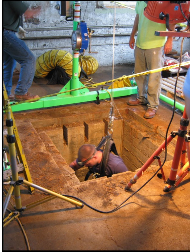
Photo 4.2: Inspector Entering Dry Wet Well
