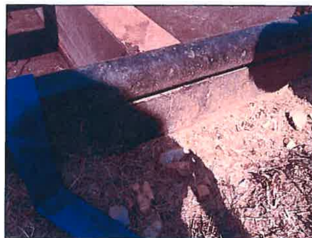
Top 6" of the aeration basin was re-enforced.
