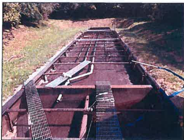
Re-enforced digester wall
