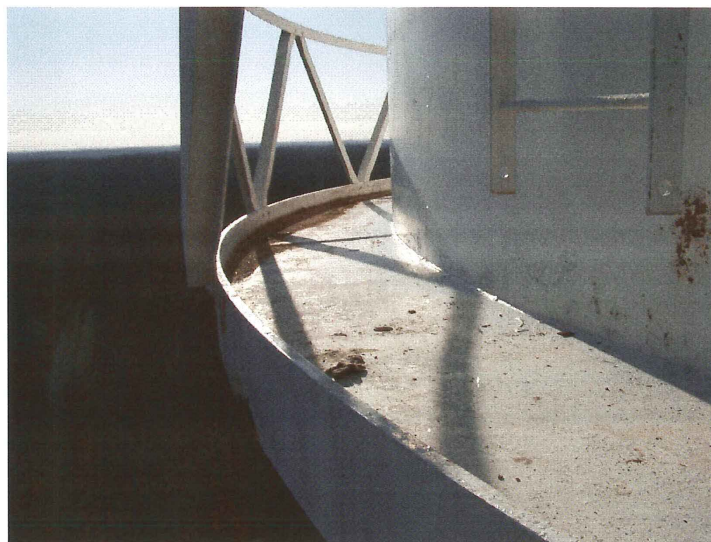
Photo shows the 4" tall kick plate along the outer edge of the balcony.
