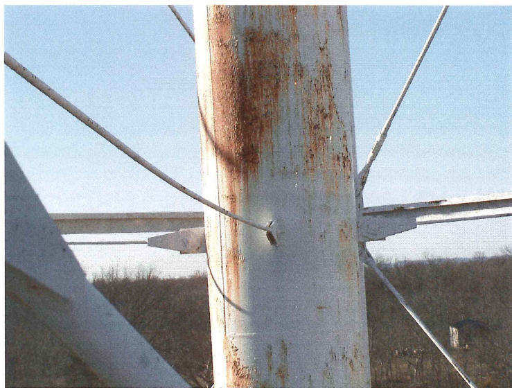
Photo shows the riser stay rods at the lower strut level. The rod connections appear sound.
