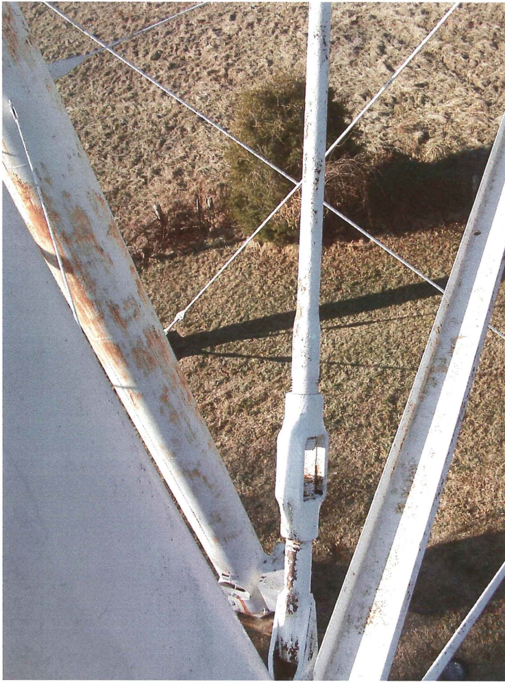
Photo shows an upper panel windage rod. All rods were properly adjusted.
