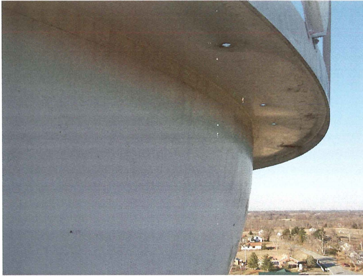
Photo shows the underside of the balcony and the upper section of the north lower knuckle. The coating continues to provide protection to the steel.
