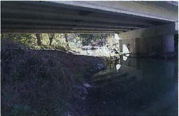
Photograph 12. Stream SKY-CDK-006, Downstream, Facing Southeast (10/15/15)
