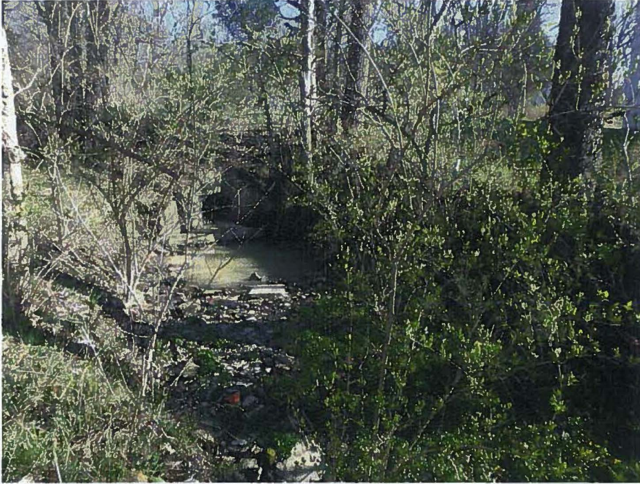
Photograph 5: Representative view of intermittent stream and culvert.
