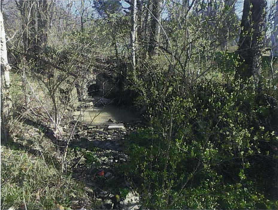
Photograph 5: Representative view of intermittent stream and culvert.
