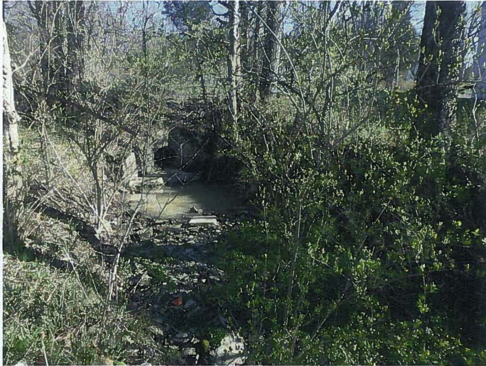
Photograph 5: Representative view of intermittent stream and culvert.
