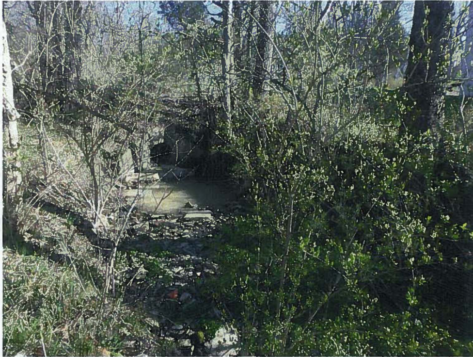
Photograph 5: Representative view of intermittent stream and culvert.
