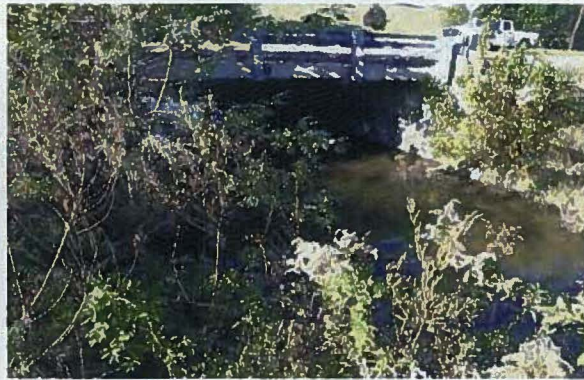
Photograph 36. Stream SKY-CDK-018, Downstream, Facing Southwest (10/16/15)
