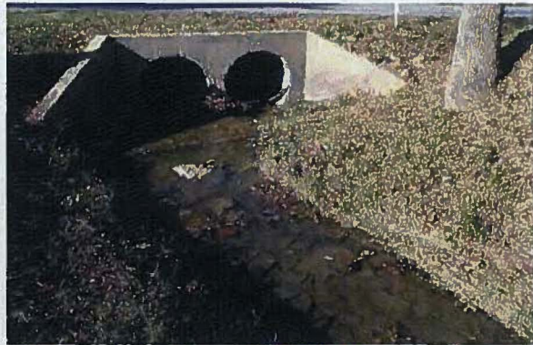
Photograph 40. Stream SKY-CDK-020, Downstream, Facing Southwest (10/16/15)
