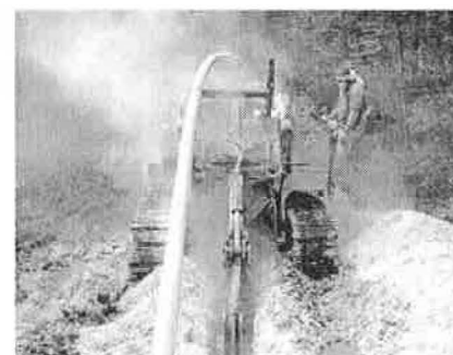
Savings from an Alliance-assisted water-loss reduction project was more than $70,000 in one year.
