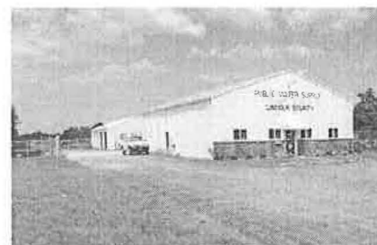
In 2010, the District switched from a commercial gas customer with Ameren to a wholesale customer through Alliance, saving $4,000 to $6,000 during the winter months on plant dehumidification and heating.
