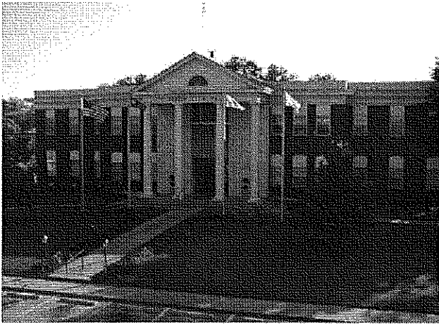
Dublin, GA, City Hall site for the Model E demonstration.
