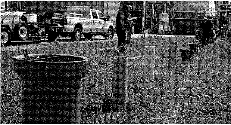
Left: Alignment of the sewer lines in the test section. Right: HDD tool crossing the sewer pipe in field tests.
