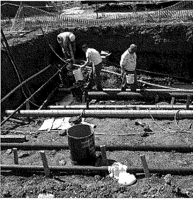
Placement of the pipes at the GTI test section.
