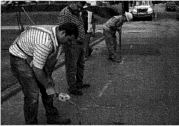
Left: Pinpointing the leak source at a cast-iron main. Right: Covering the leak area and using the Hi-Flow device to measure the gas leak rate.
