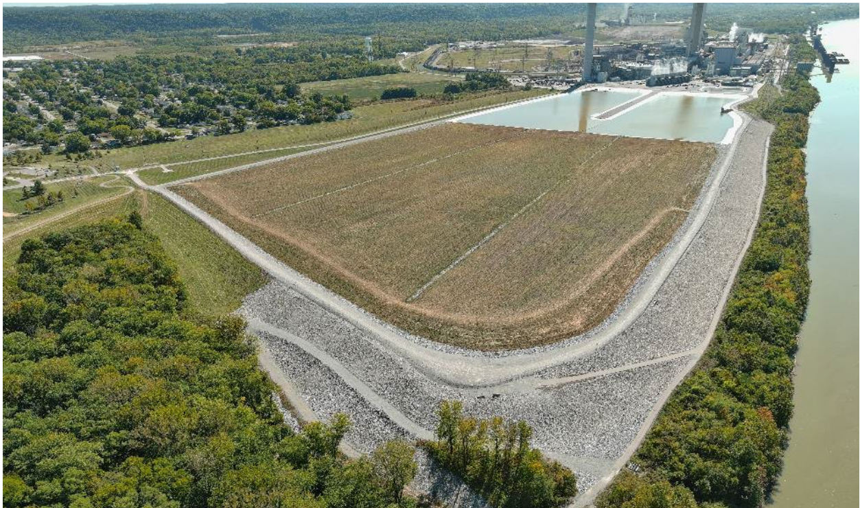
Mill Creek Main Ash Pond Closure – October 2022
