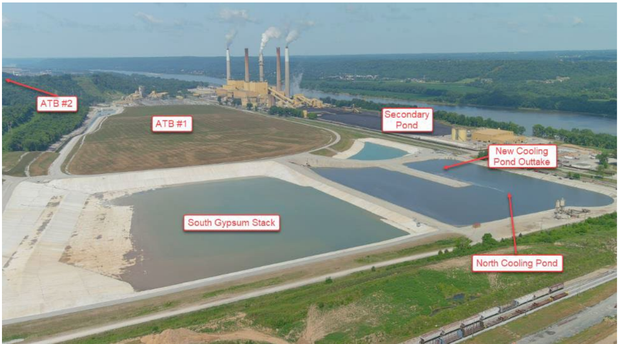
Phase II Ghent ATB #1 – Looking West – July 2022
