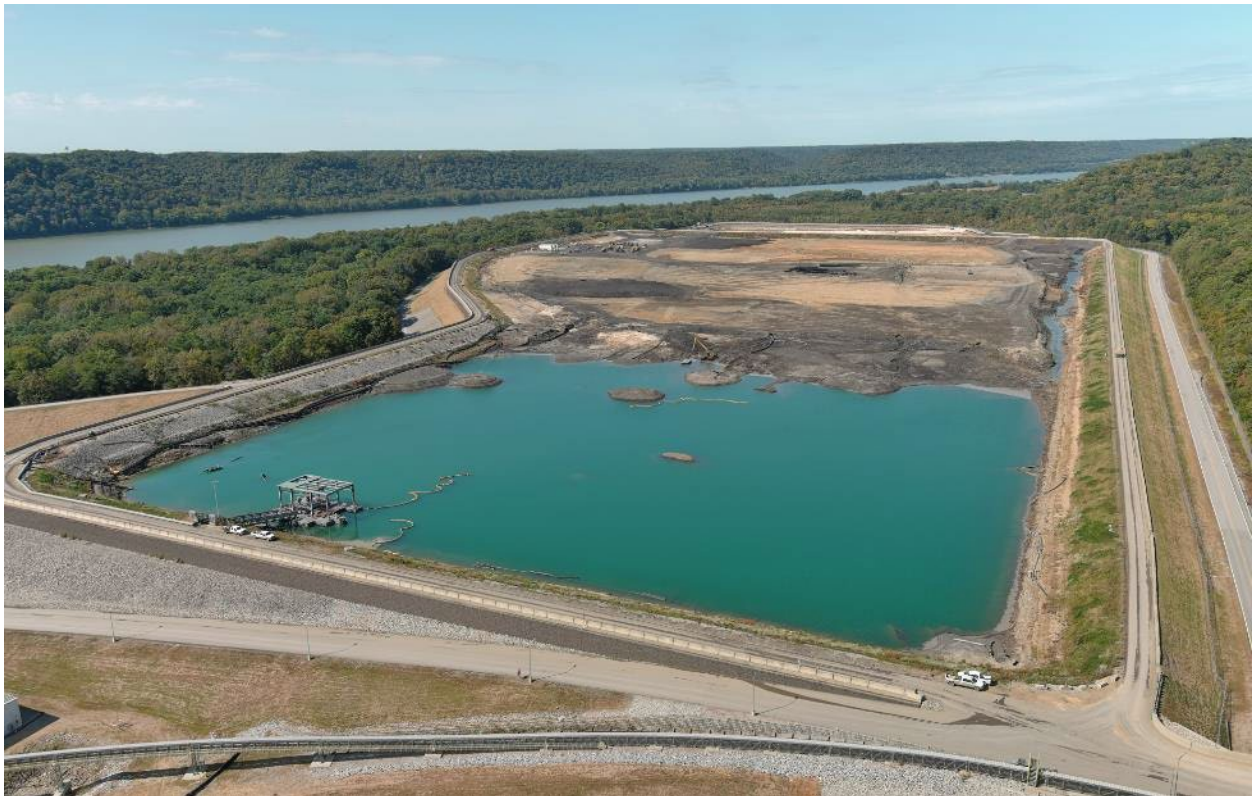
Trimble BAP – Looking North – October 2022
