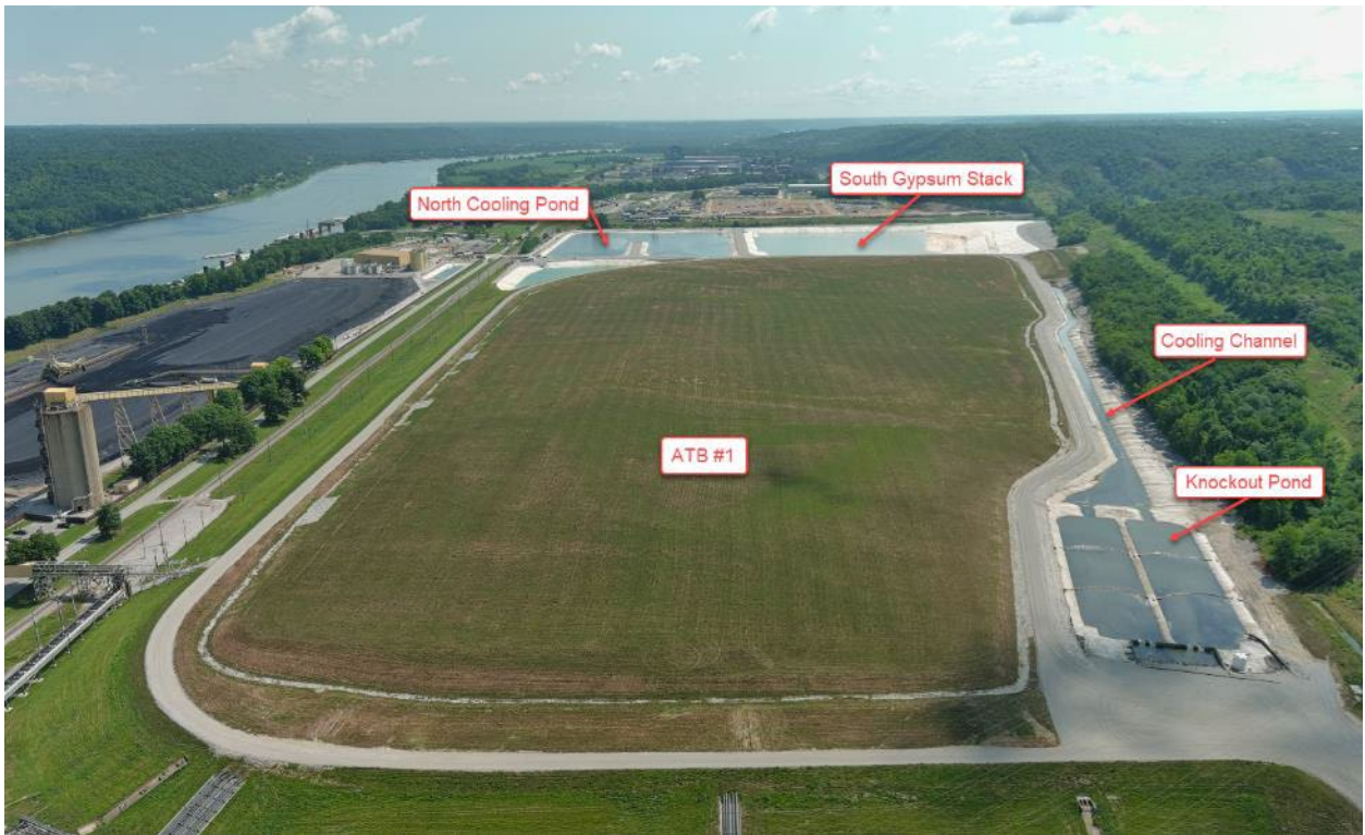
Phase II Ghent ATB #1 and Cooling Channel – Looking East – July 2022
