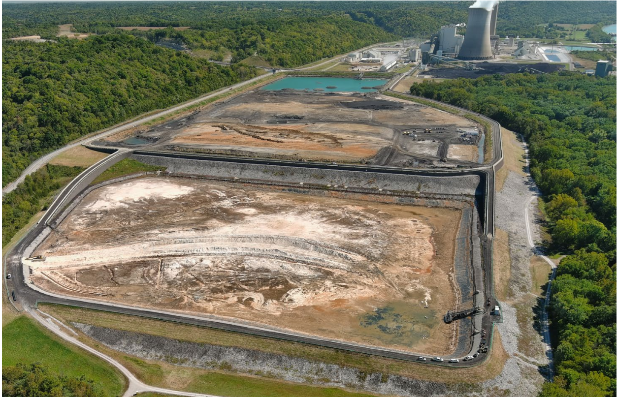
Trimble GSP – Looking South – October 2022
