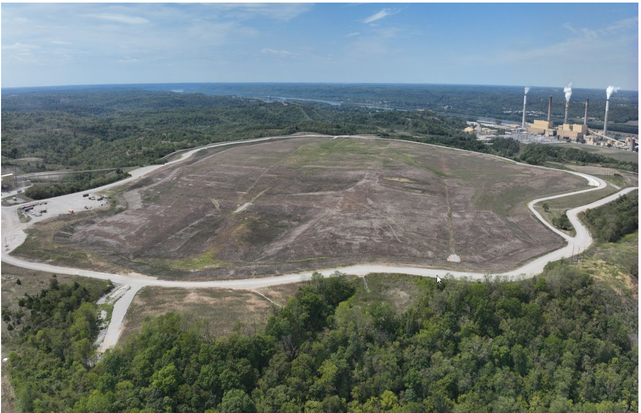
Phase III Ghent ATB #2 – September 2024
