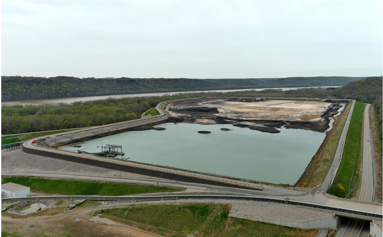
Trimble BAP – Looking North – April 2023
