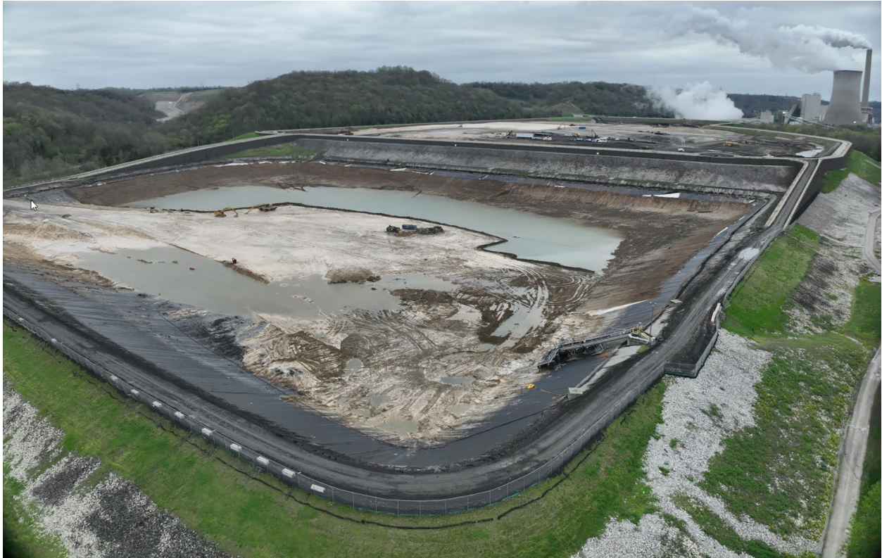
Trimble GSP – Looking South – March 2024
