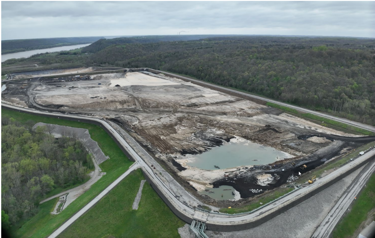
Trimble BAP – Looking Northeast – March 2024
